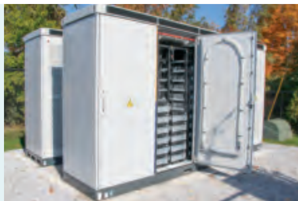
Lithium-ion battery during installation
