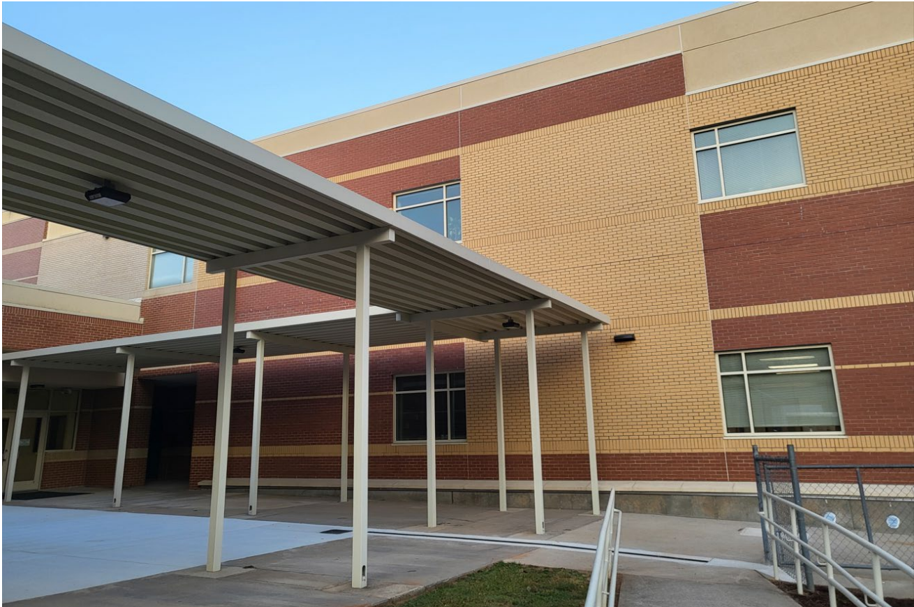
Source: Taken by MGT staff during the onsite visit.
