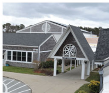
Nauset Regional School District House Doctor Contract
