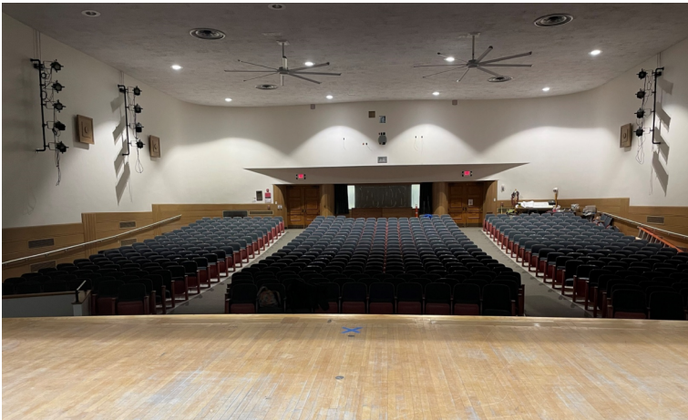
WBS - Auditorium Final Cleaned New Lighting & Fans
