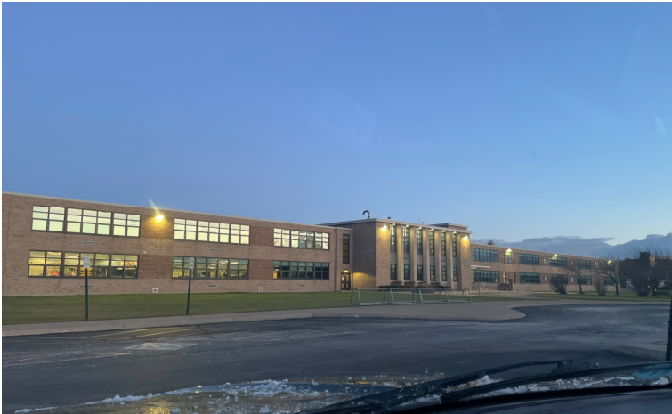
WBS - Building Exterior New Wall Mounted Lighting
