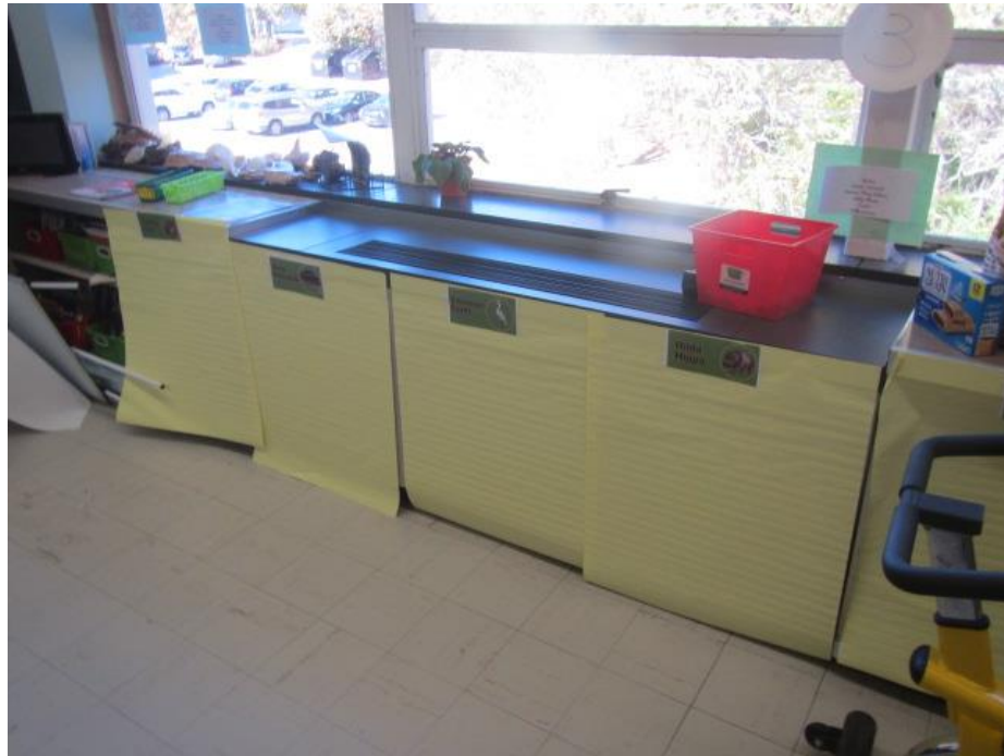
Univent return vent (bottom front) obstructed by paper preventing airflow into unit
