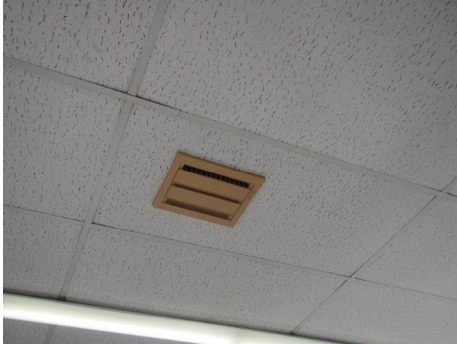
Abandoned vent in ceiling of Teacher's Room (possible former smoking vent)
