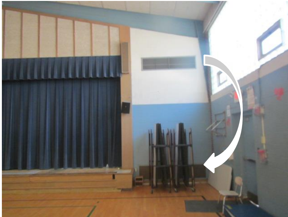
Short-circuiting of AHU in gymnasium, arrow shows airflow
