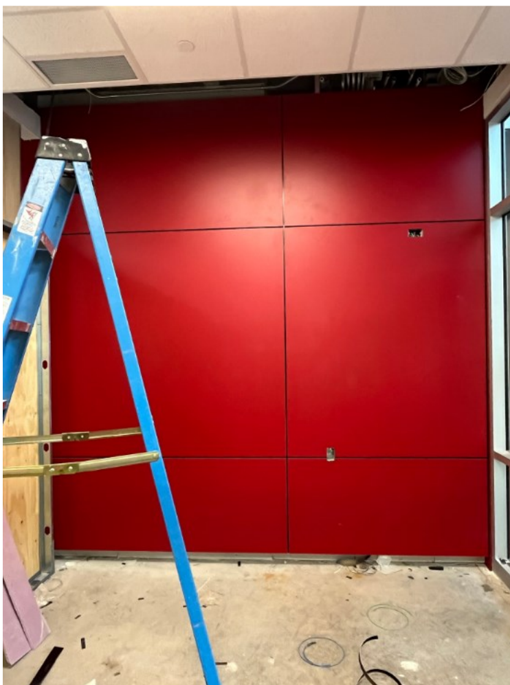
From top left: New flooring in administrative addition; new light fixtures in west hallway; wall tile in new breakroom; phenolic panels in new front entry; phenolic panels for the exterior (December 2024)
