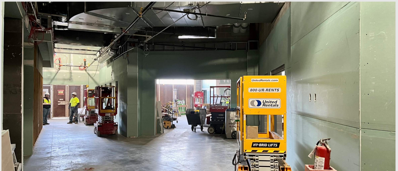
Below: a view of the progress in the River Bluff addition entrance and corridor space as drywall tape & finish begins
