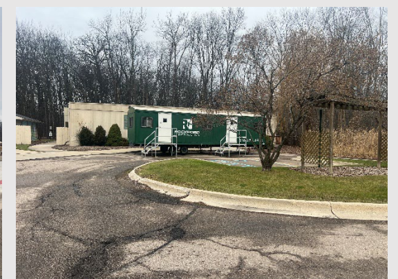
Bingham Farms - Construction Trailer
