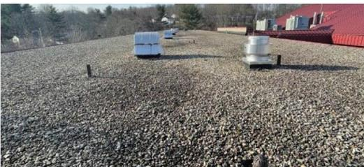
Pictured Above: The 1958 wing of Slade Middle School has a 1.5" metal deck roof with pearl-lite insulation. The roof then has pond stones on it to promote drainage through a system of roof drains and gutters
