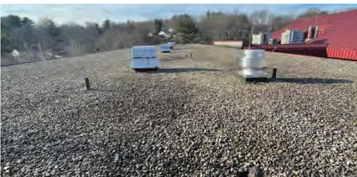
Pictured Above: The 1958 wing of Slade Middle School has a 1.5" metal deck roof with pearl-lite insulation. The roof then has pond stones on it to promote drainage through a system of roof drains and gutters
