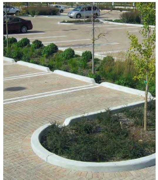
Parking lot bioswales and pervious paving
