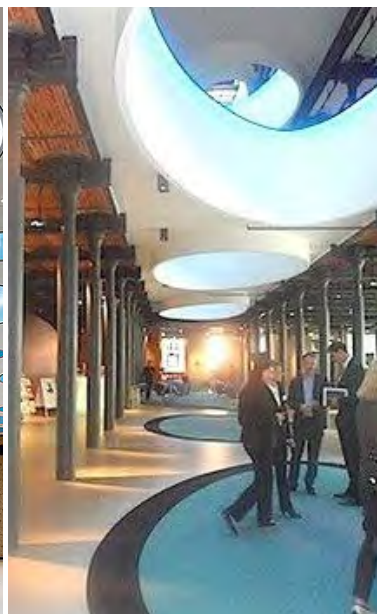
Light tubes, operable skylights and vertical openings through the buildings to provide natural light and ventilation to the center of buildings
