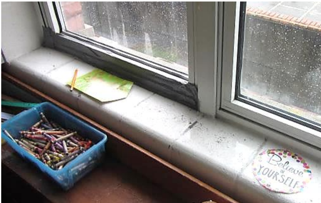
Standing water from active leak on masonry/windowsill in classroom 215, note duct tape on left window
