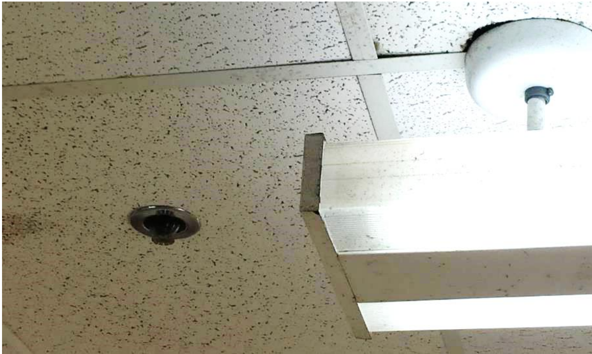
Dust/debris/staining on light fixture directly in front of univent, also note sprinkler head
