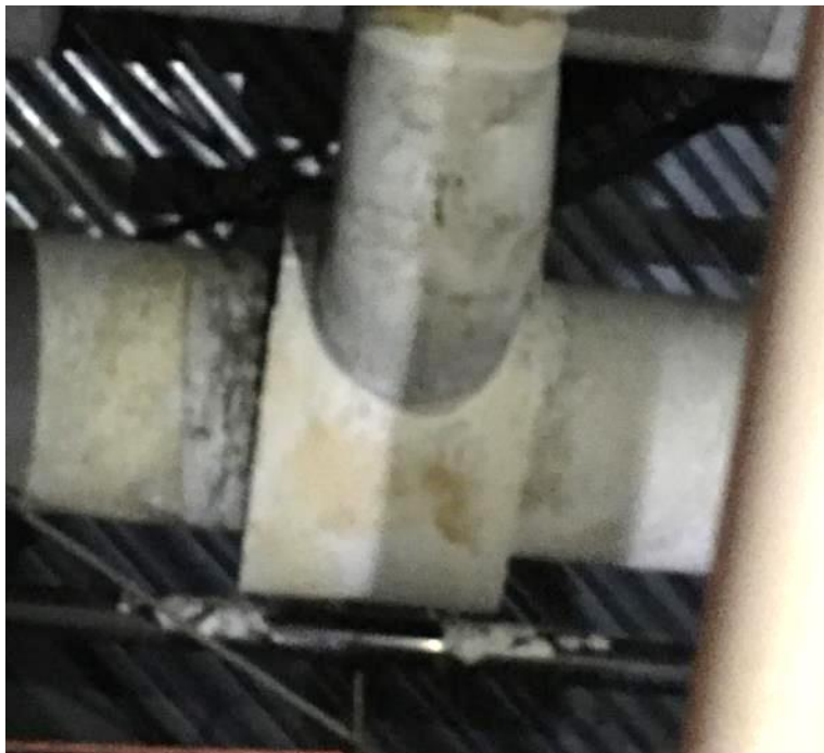
Insulation material in art room closet
