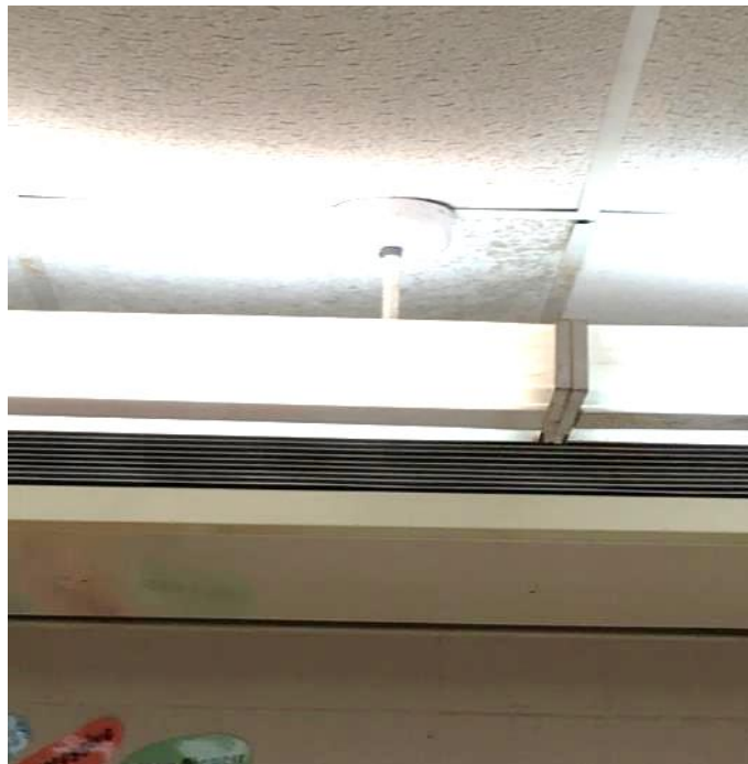
Suspended lighting fixture and stained tile in front of univent
