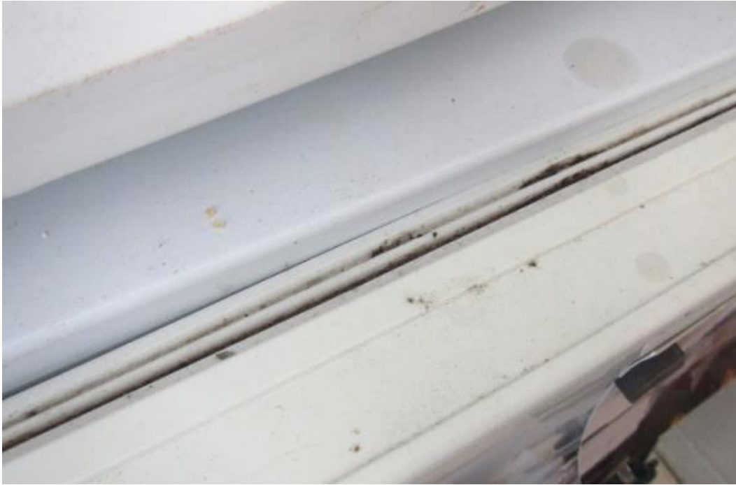
Debris/mold growth on mini-fridge gasket in classroom
