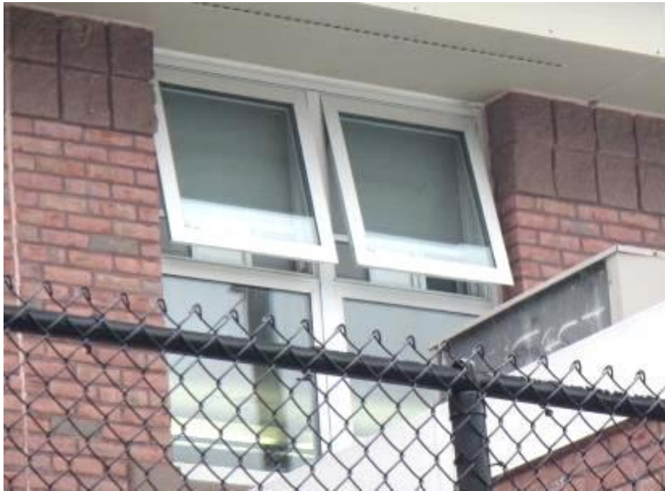
Classroom windows open while AC system in operation
