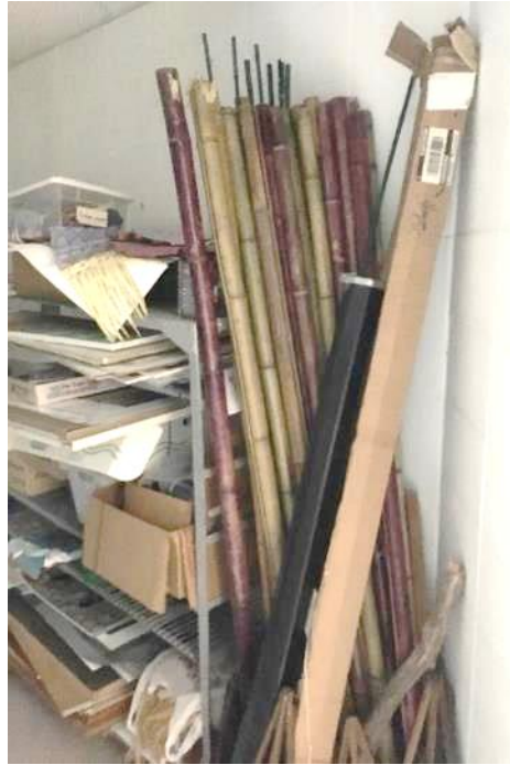
Moldy/odorous bamboo in Art room closet
