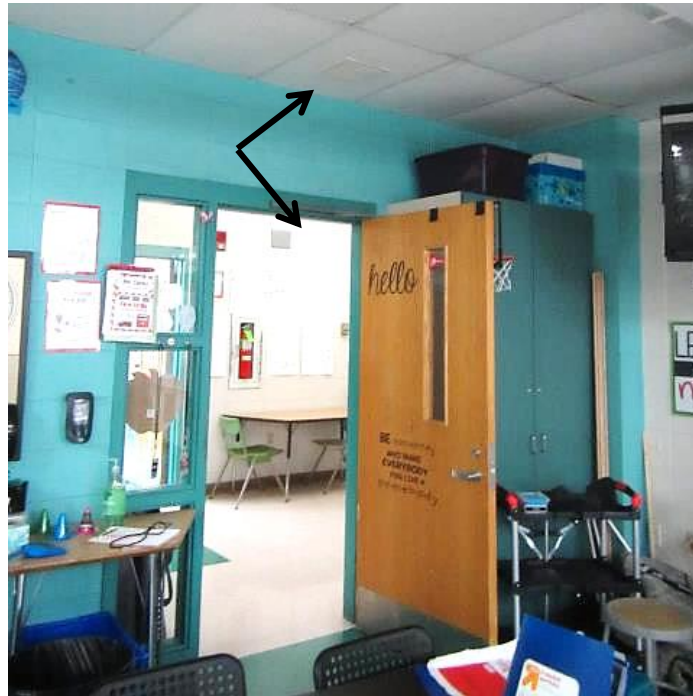
Proximity of classroom exhaust vent (arrows) to open hallway door
