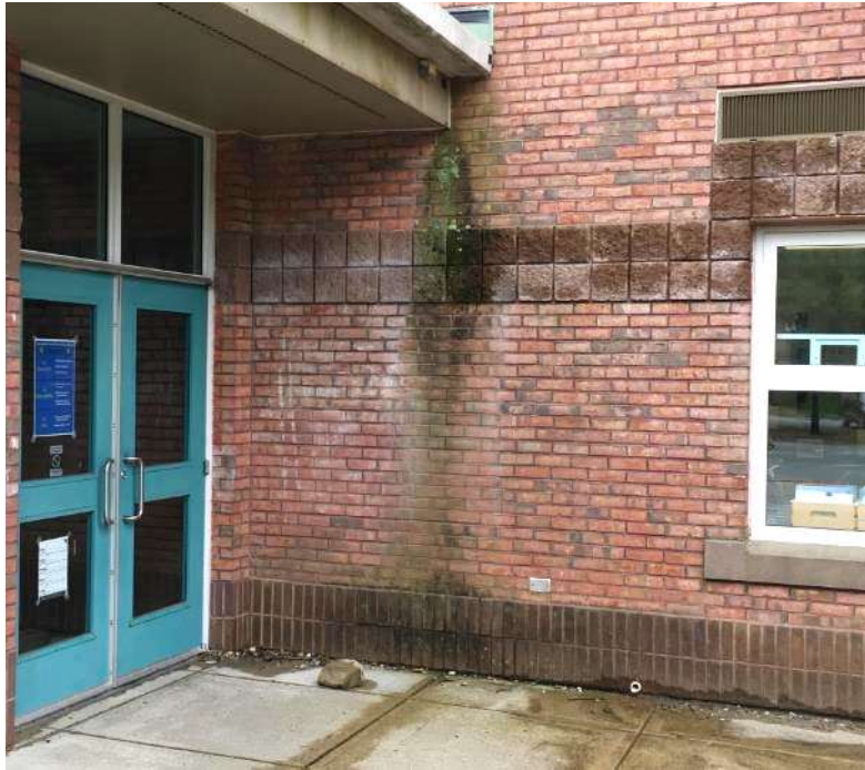
Moss growth from chronic water exposure on exterior walls
