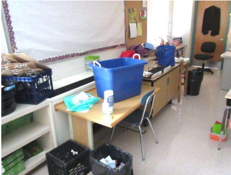
Univent return vent (bottom front) obstructed by classroom furniture
