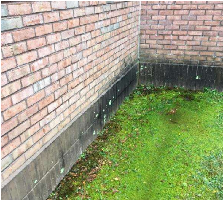
Heavy moss growth/discoloration of foundation due to chronic water exposure (i.e., splash back) from lack of drainage/gutters/downspouts
