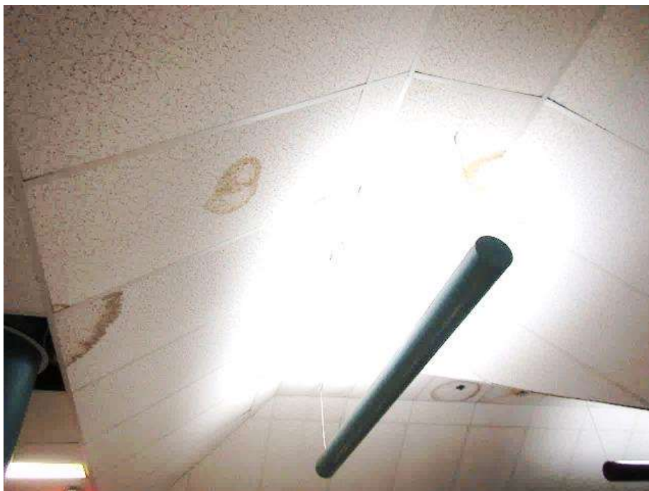
Water-damaged ceiling tiles in 2 nd floor hallway near Room 217
