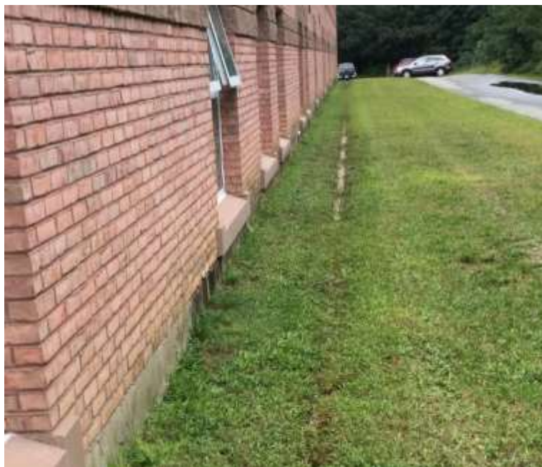
Trough along exterior of building due to roof runoff/lack of gutters, also note open classroom window while AC system operating
