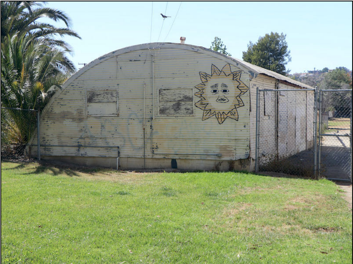
Photo 10. Quonset Building, viewed from south. [5-24-21]
