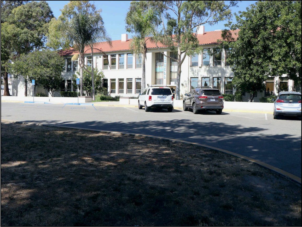
Photo 1. Main School Building, western elevation, viewed from southwest. [5-24-21]
