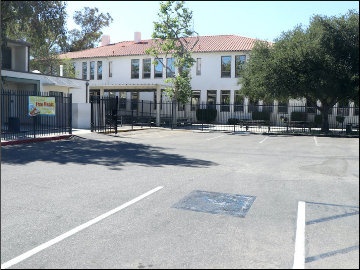
Photo 5. Main School Building, southern wing, viewed from south. [5-24-21]
