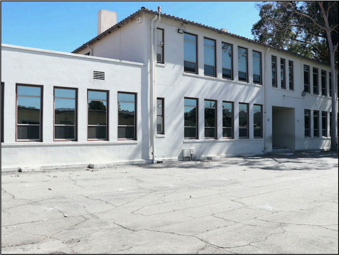
Photo 3. Main School Building, northern wing, viewed from north. [5-24-21]
