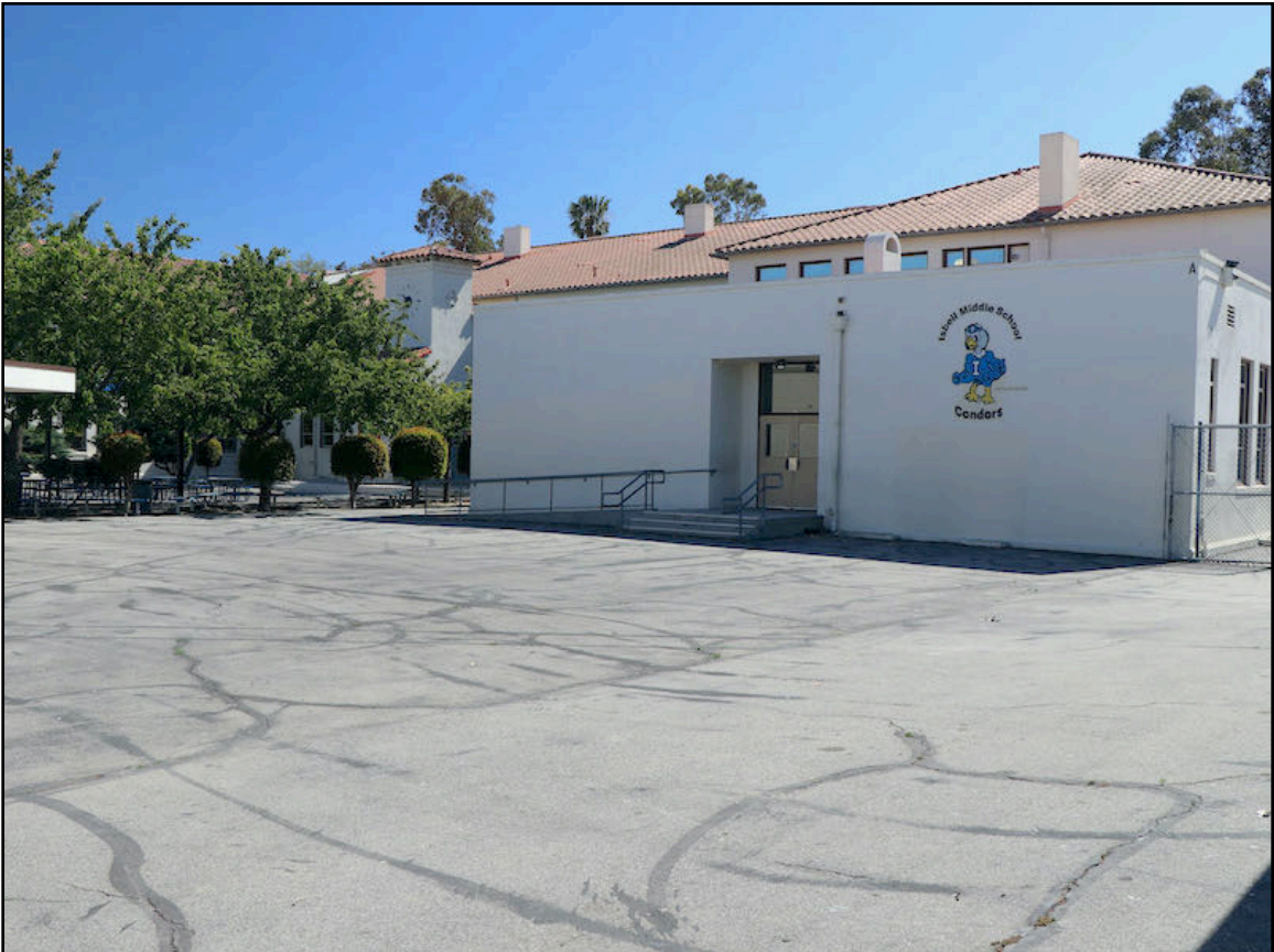
Photo 2. Main School Building, eastern elevation, viewed from northeast. [5-24-21]
