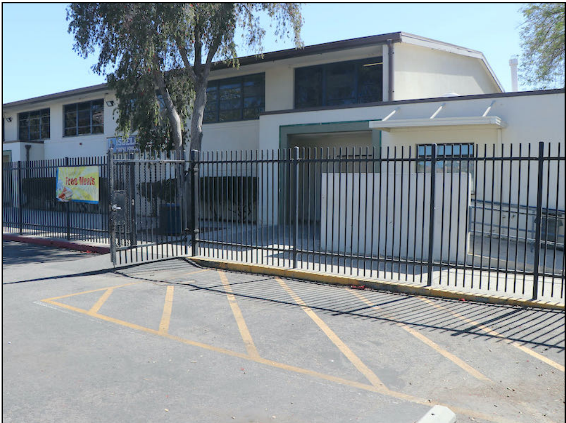
Photo 8. Cafetorium Building, eastern elevation, viewed from northeast. [5-24-21]
