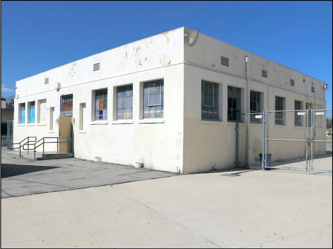
Photo 6. Manual Arts Building, western and southern elevations, viewed from southwest. [5-24-21]
