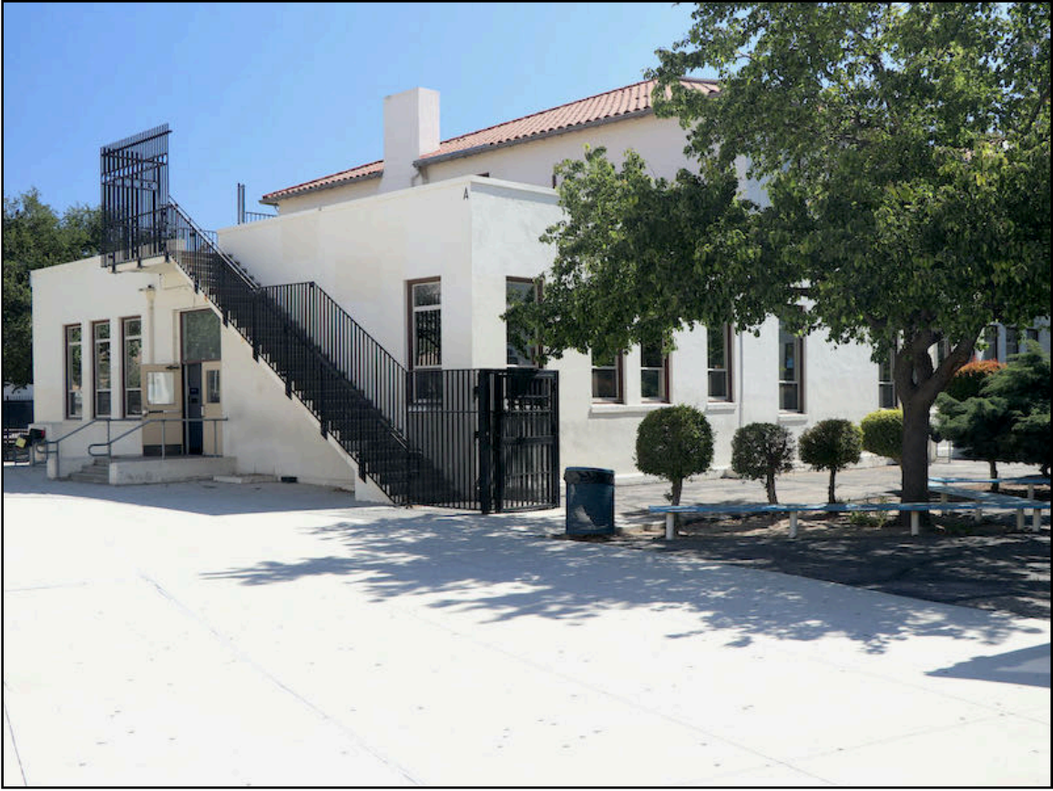
Photo 4. Main School Building, southern wing, viewed from northeast. [5-24-21]
