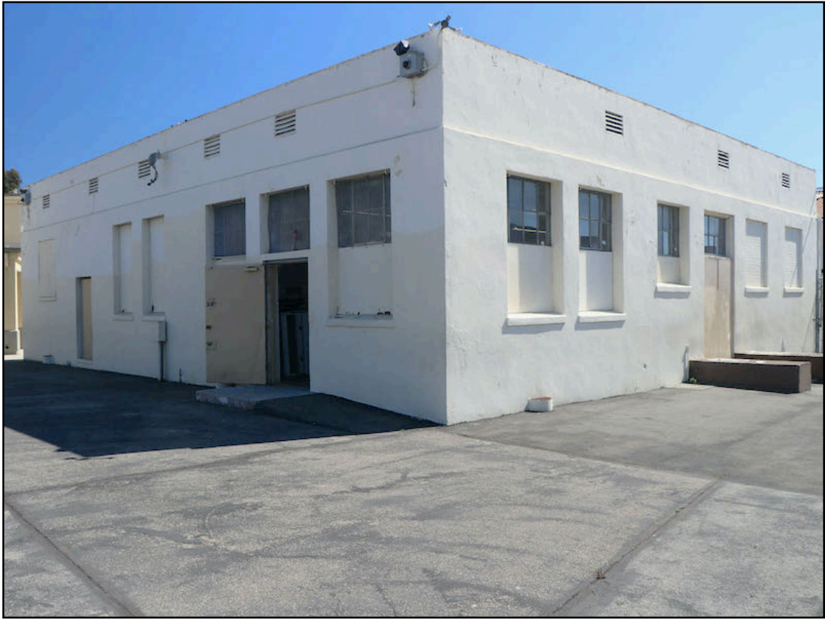
Photo 7. Manual Arts Building, eastern and northern elevations, viewed from northeast. [5-24-21]
