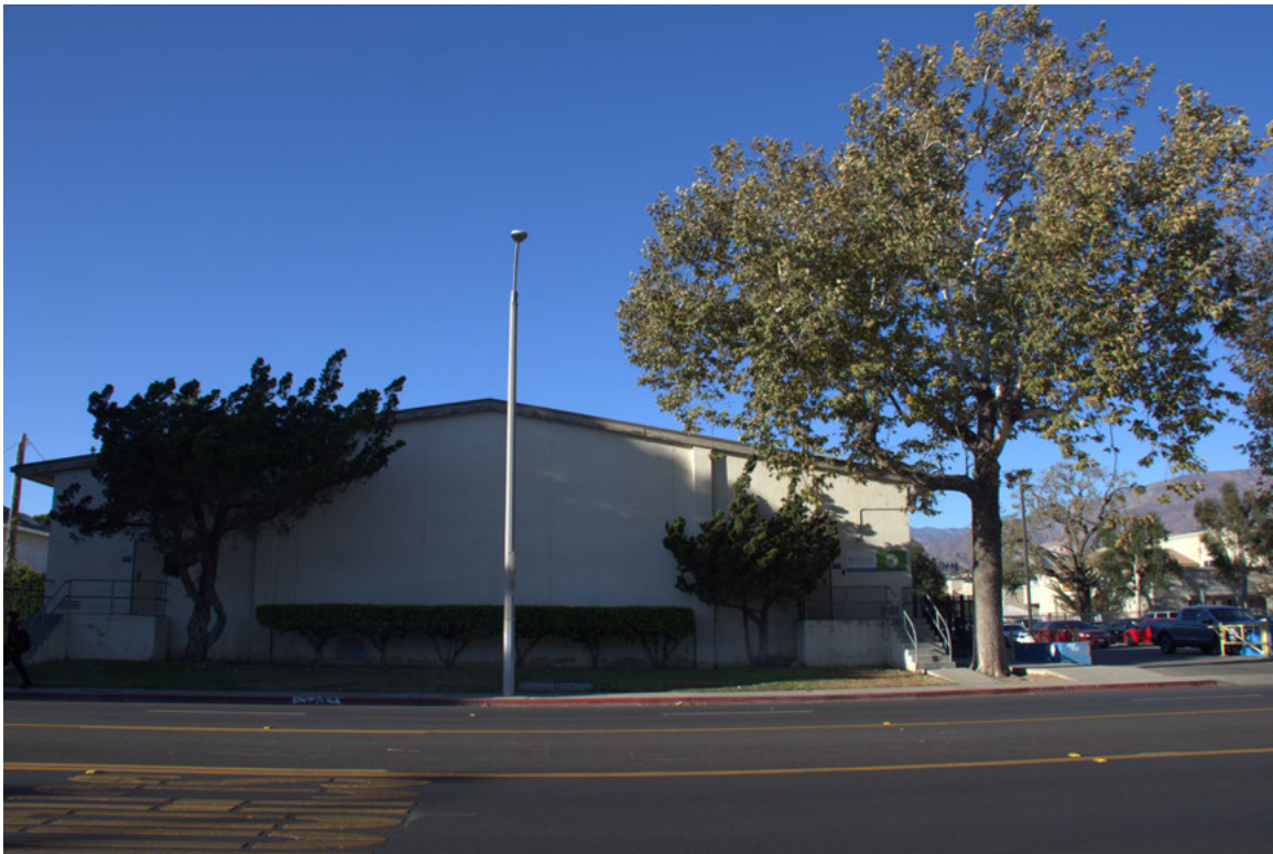
View of cafeteria building from Harvard Boulevard, looking north.
