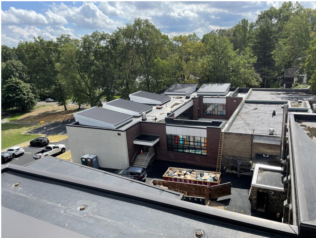
Delia Bolden (Jefferson ES) New Wing Addition
