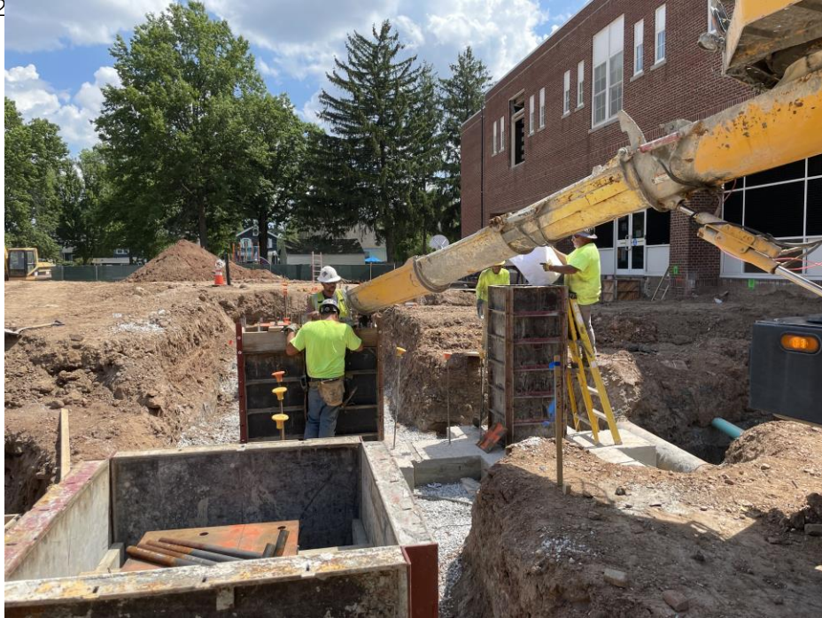
New Footings/ Piers Area B - Clinton Elementary School
