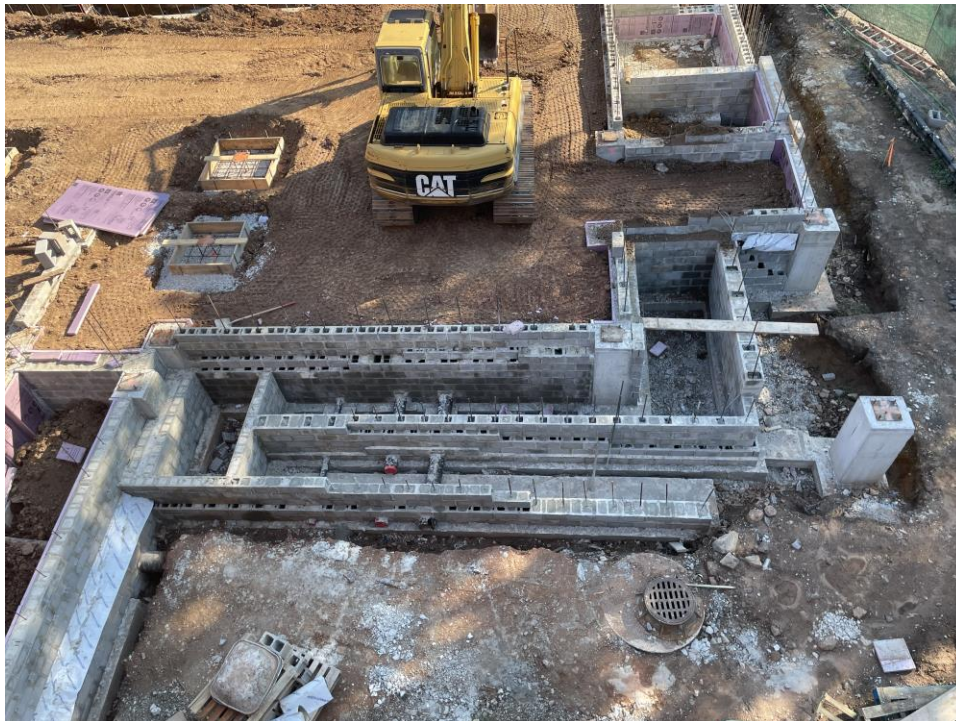
New Ramp at Area B- New Wing Addition
