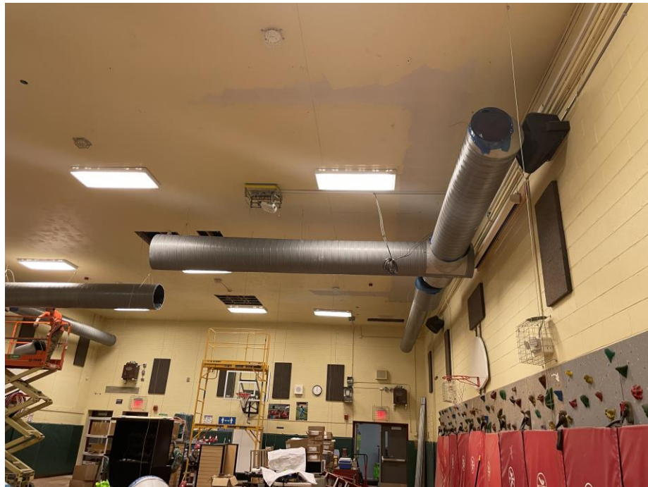
New Spiral Ductwork at Gym - Clinton Elementary School
