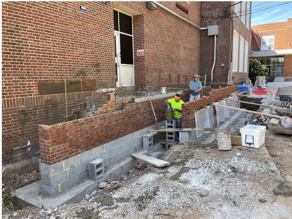
Brick on new Ramp at Cafeteria - Clinton Elementary School
