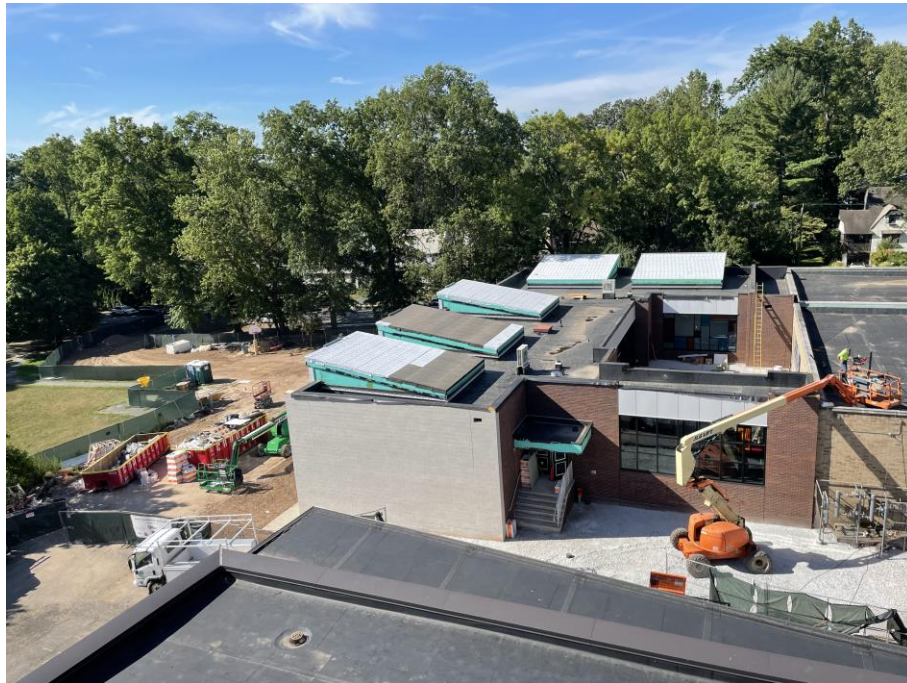
Contractor finishing around exterior - Jefferson Elementary School
