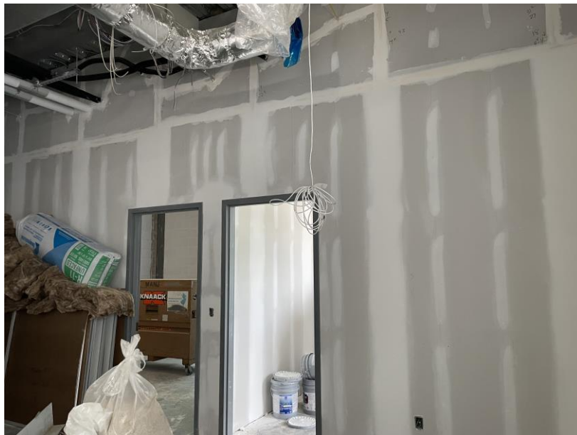
Tape and spackle at new office area - Clinton Elementary School
