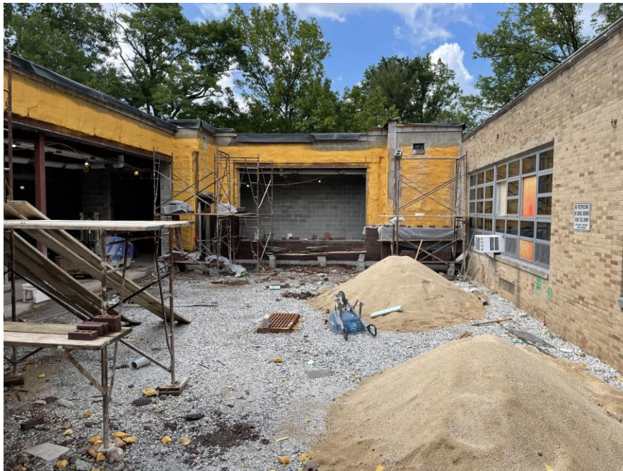
Courtyard new brick installation - Jefferson Elementary School
