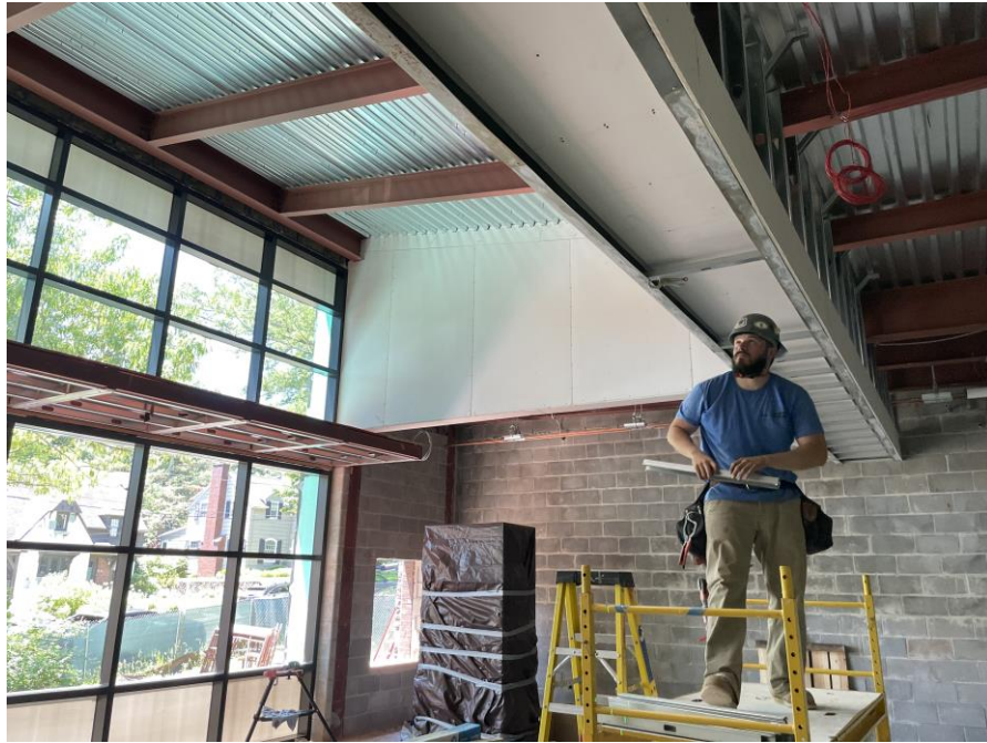
Contractor framing interior of building - Jefferson Elementary School
