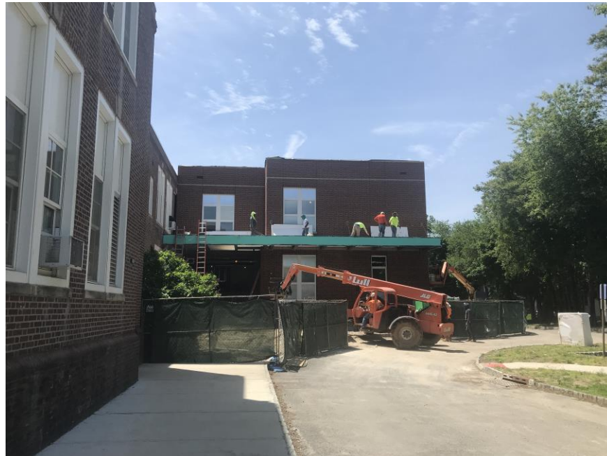
Canopy Entrance Roof underway - Clinton Elementary School
