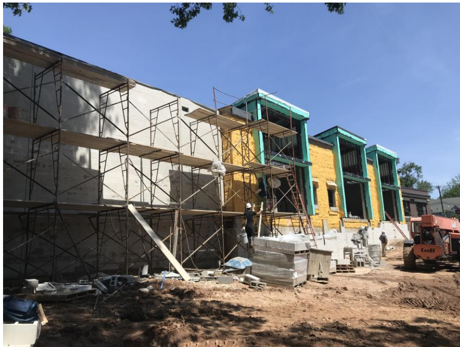
Glazed Block at exterior wall - Jefferson Elementary School
