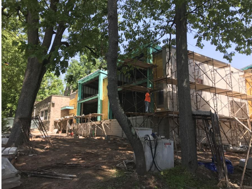
Power washing at exterior block - Jefferson Elementary School
