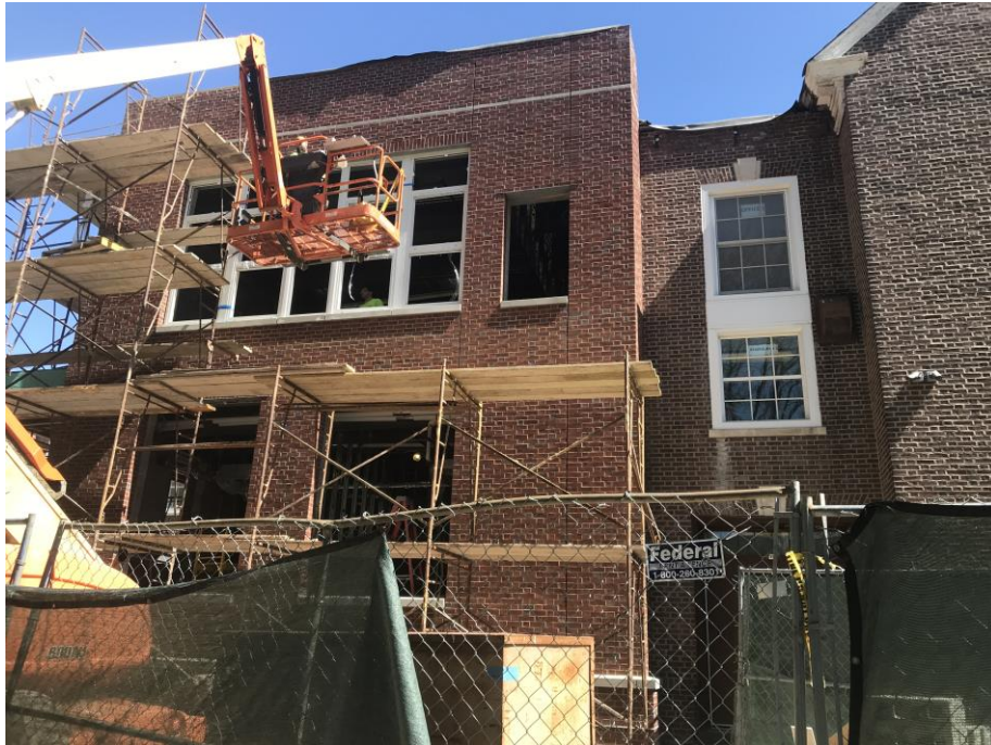
Window installation underway- Clinton Elementary School
