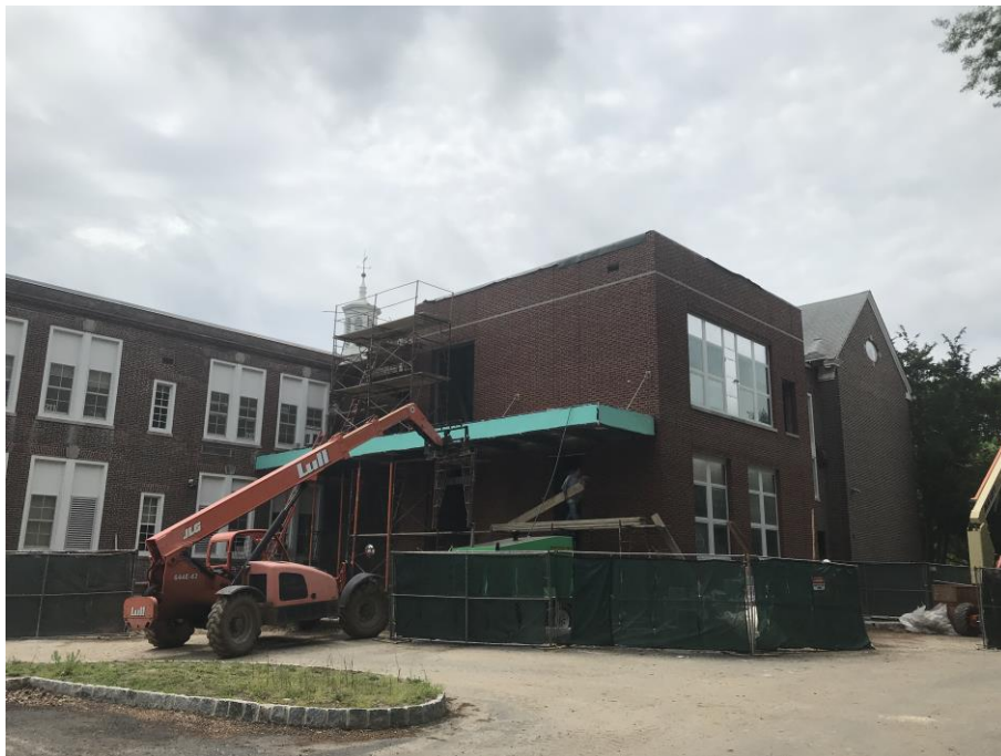
Finishing brick veneer at Area A - Clinton Elementary School
