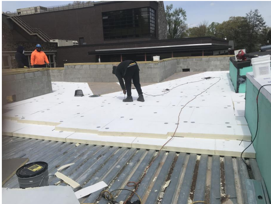
Roof work underway - Jefferson Elementary School
