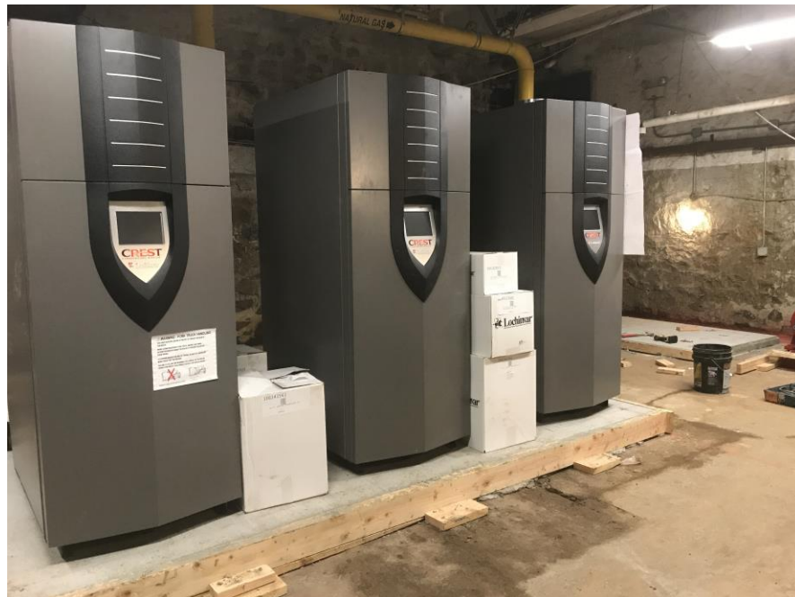
New Boilers setting underway - Jefferson Elementary School
