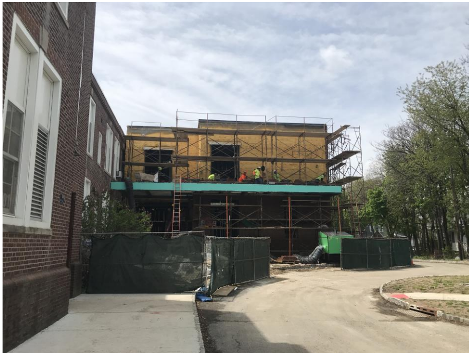
Brick veneer installation at Area A - Clinton Elementary School
