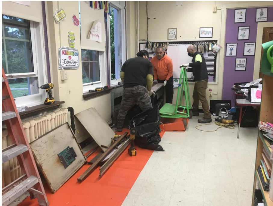
Old Unit Ventilator removals underway- Clinton Elementary School
