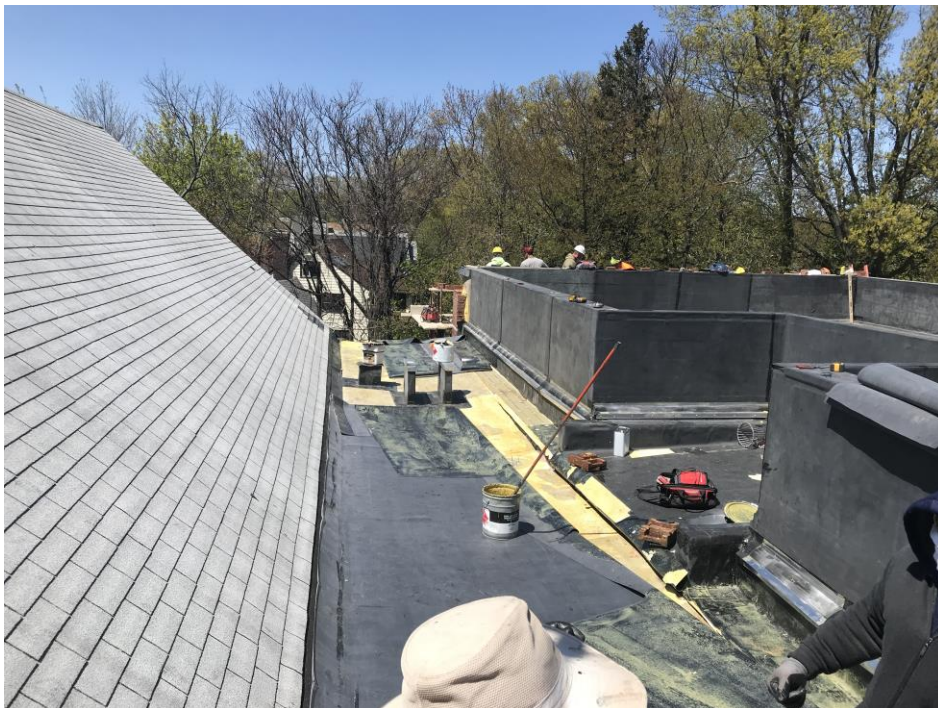
Roofing underway at Area A - Clinton Elementary School
