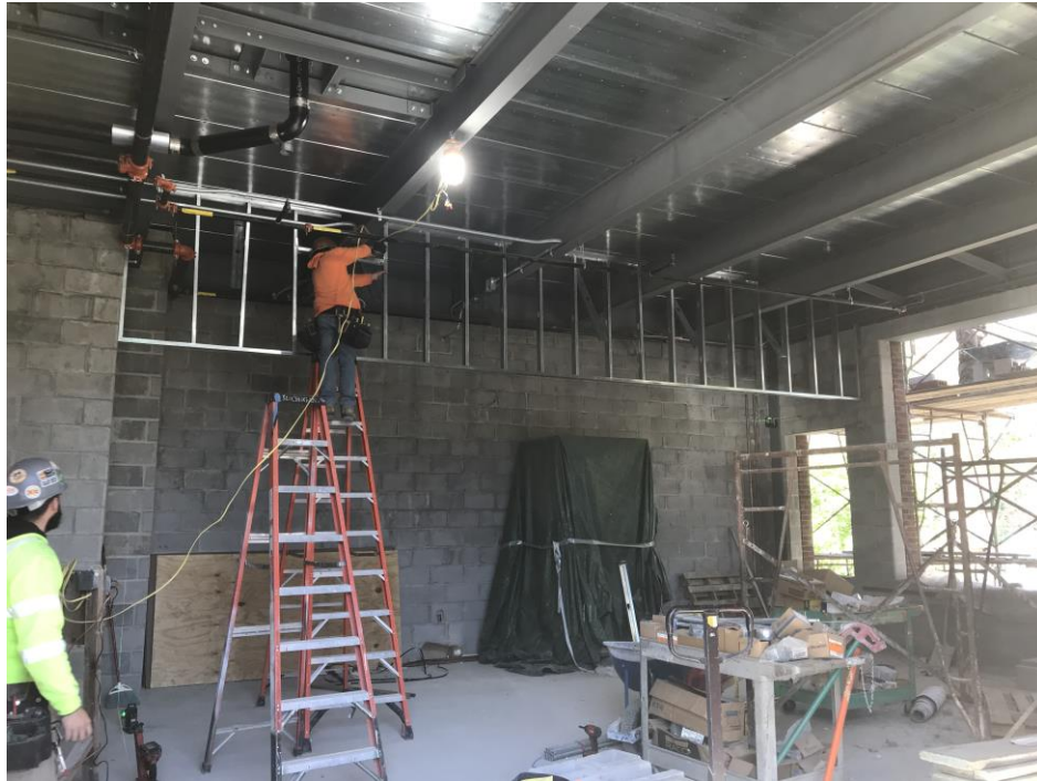
Interior Framing underway- Clinton Elementary School
