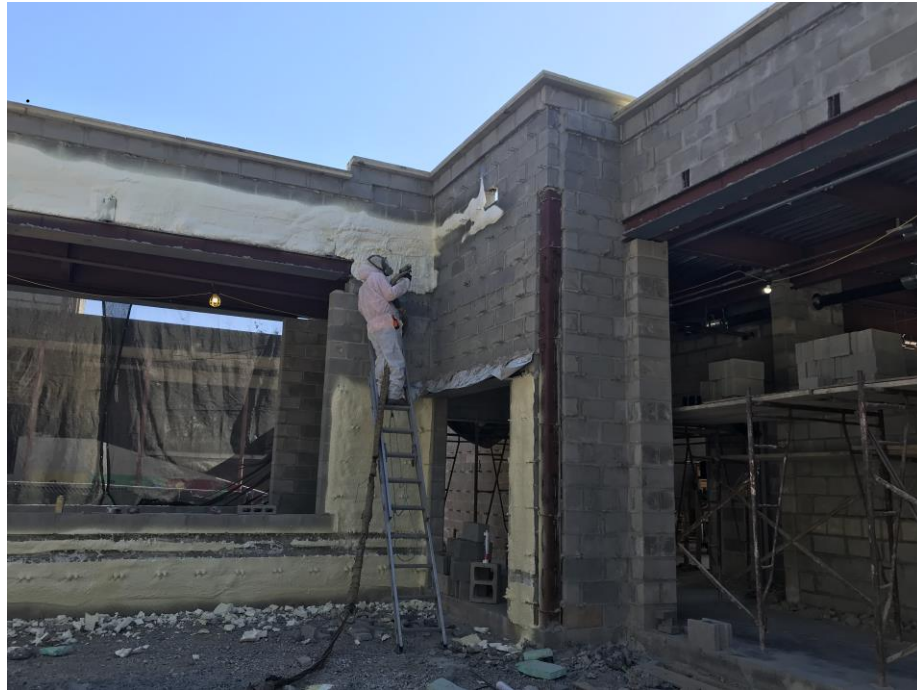
Spray on Insulation underway - Jefferson Elementary School
