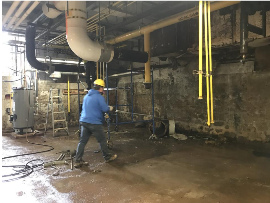
Boiler demolition underway - Jefferson Elementary School
