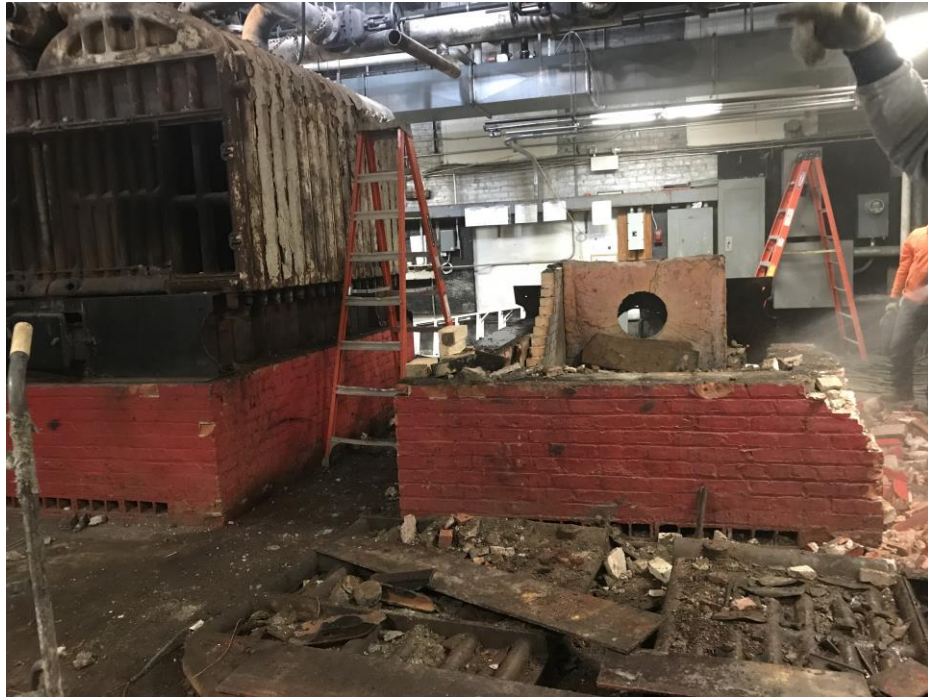
Boiler Demolition underway- Clinton Elementary School
