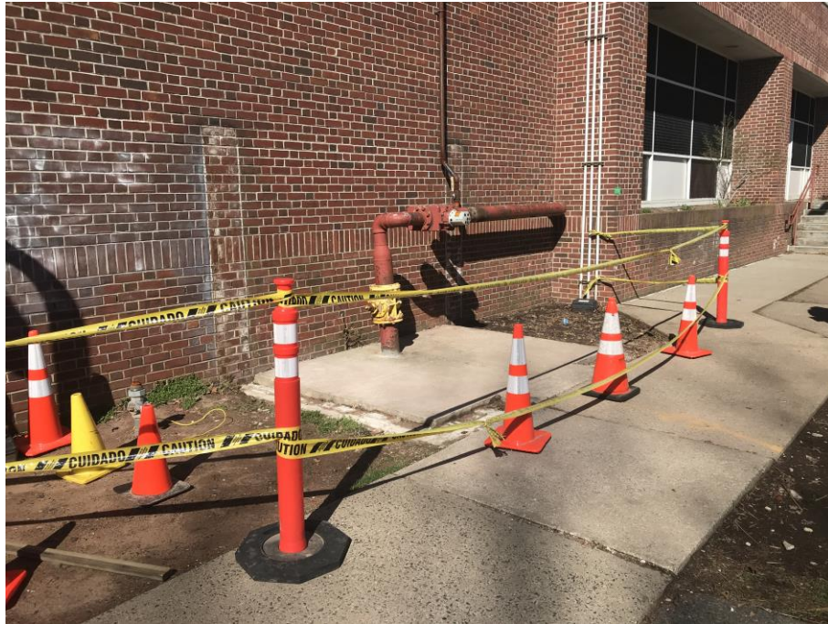
Demolished Brick Enclosure around existing gas meter - Clinton Elementary School
