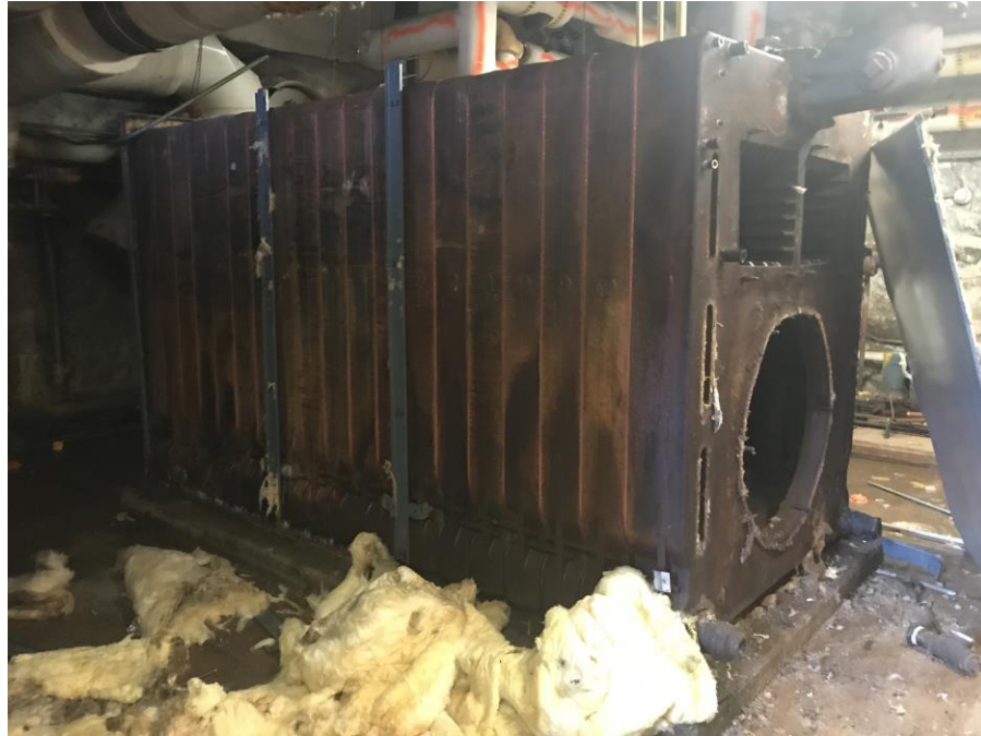
Boiler demolition underway - Jefferson Elementary School
