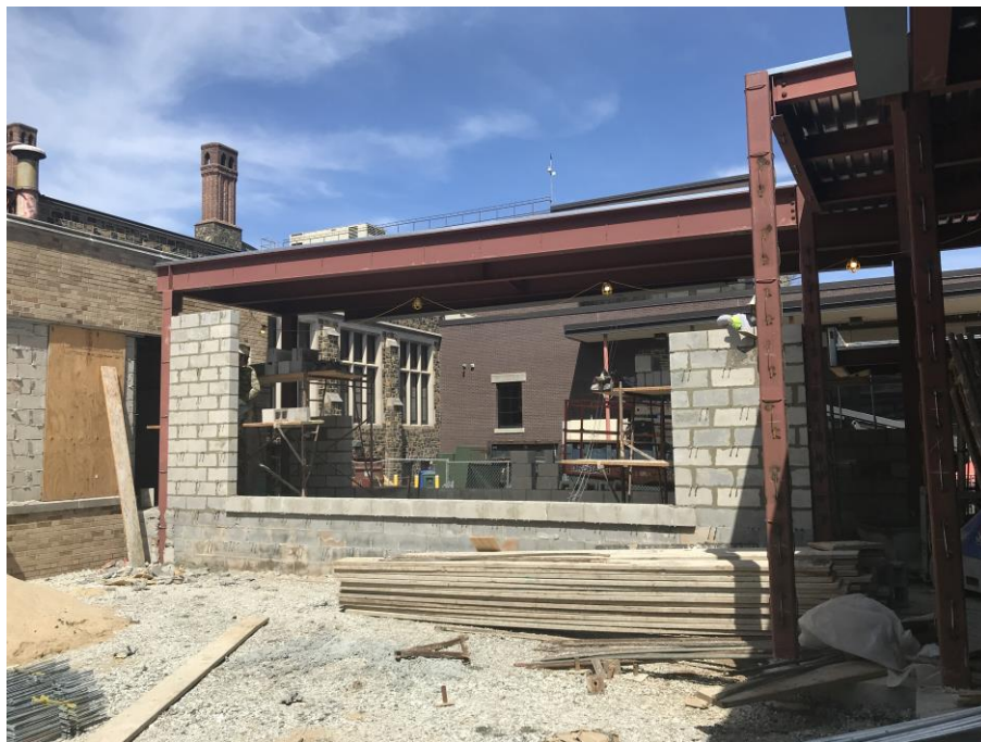
Masons working on exterior wall - underway - Jefferson Elementary
