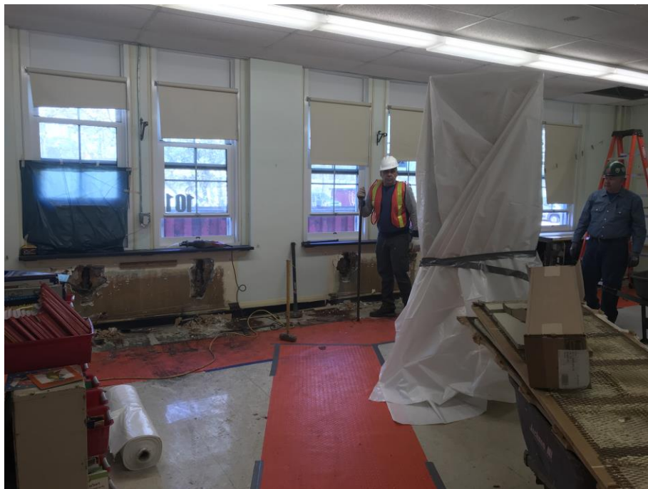
HVAC demolition at room A101 - Clinton Elementary School
