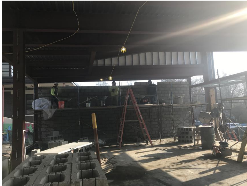
Masons working on CMU exterior wall - Jefferson Elementary School
