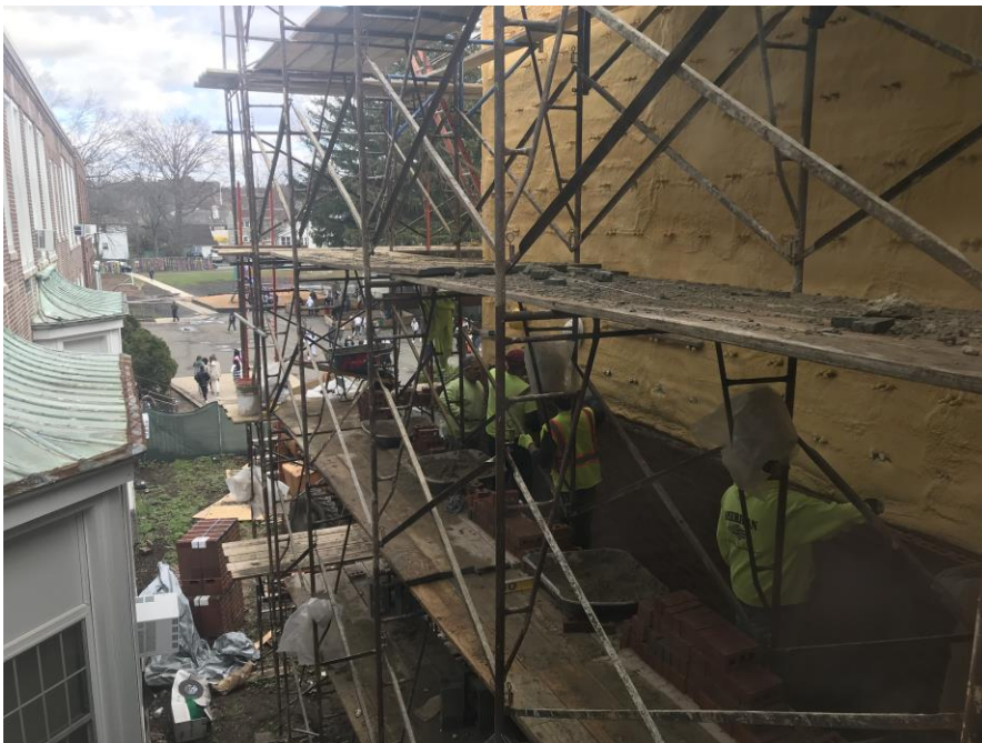
Continued with Brick wall at Area C underway - Clinton Elementary School
