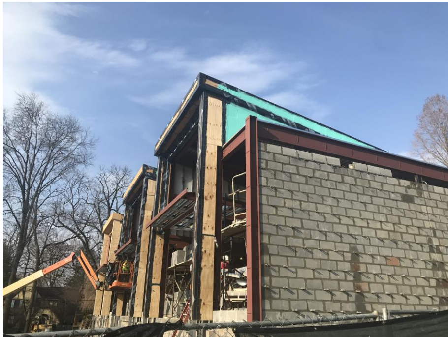
Carpenter at exterior columns underway - Jefferson Elementary
