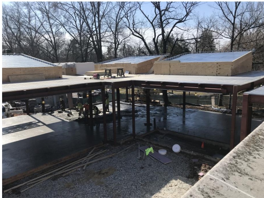
Pouring slab on grade - Jefferson Elementary School
