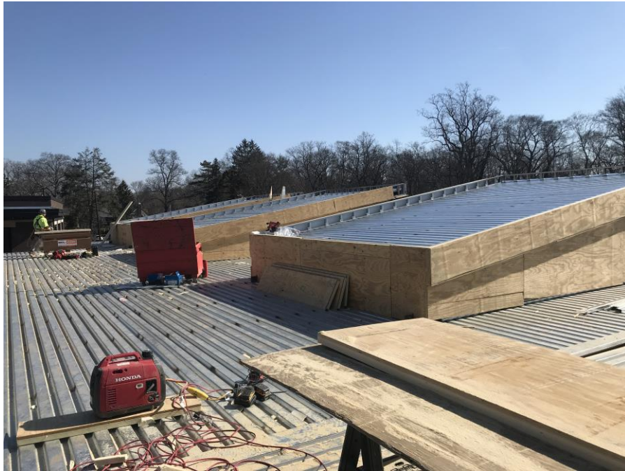
Continued with metal framing and plywood - Jefferson Elementary School
