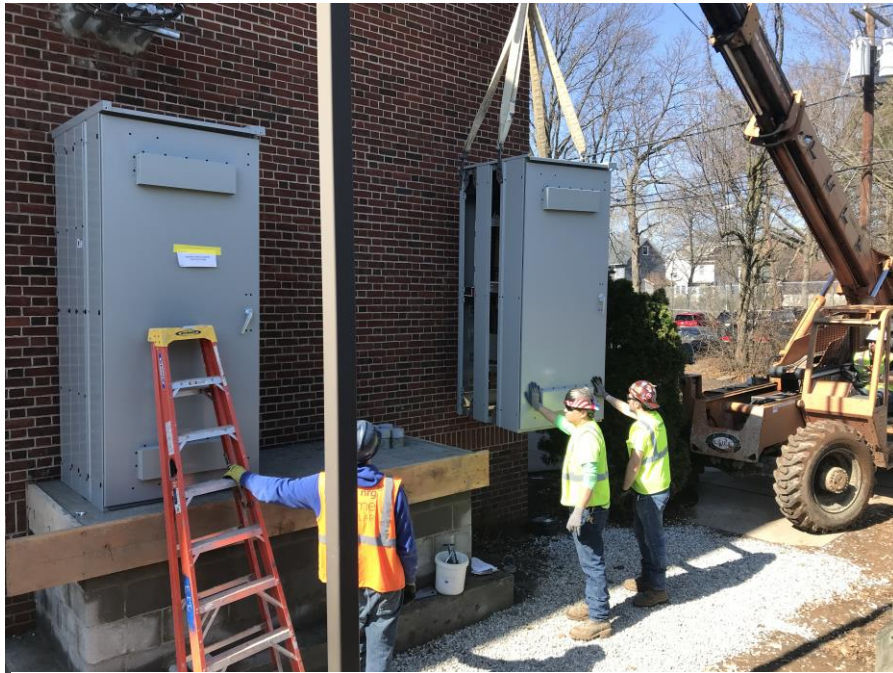
New Switchgear mounting underway - Clinton Elementary School
