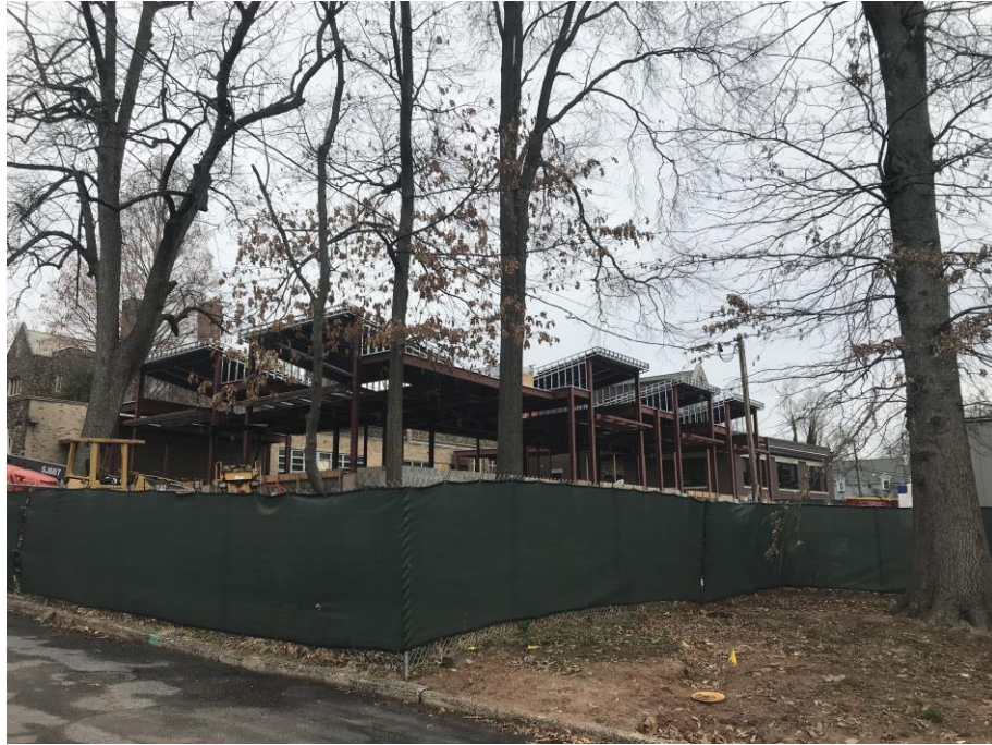
Roof metal welding framing underway - Jefferson Elementary School
