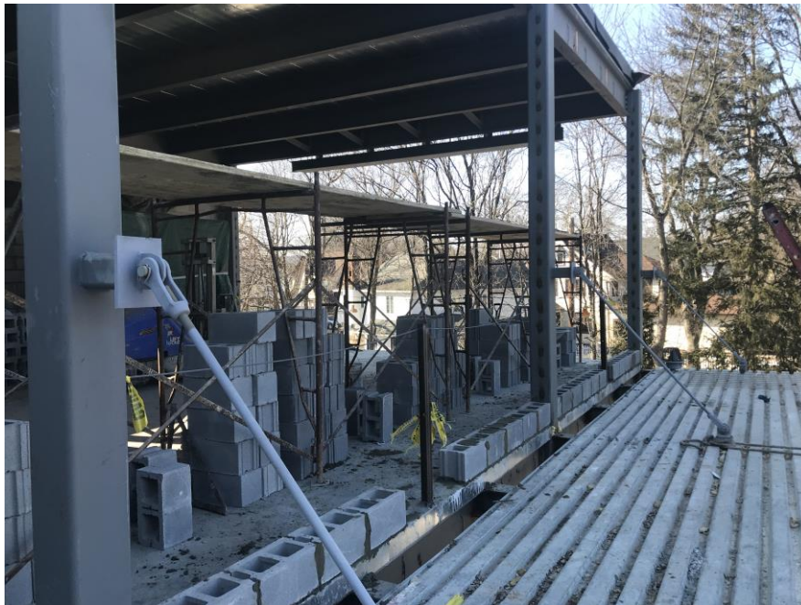
CMU Block at Second floor area A - Clinton Elementary School
