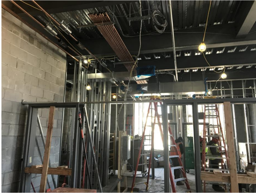
Framing, ductwork, sprinkler piping underway - Clinton Elementary School
