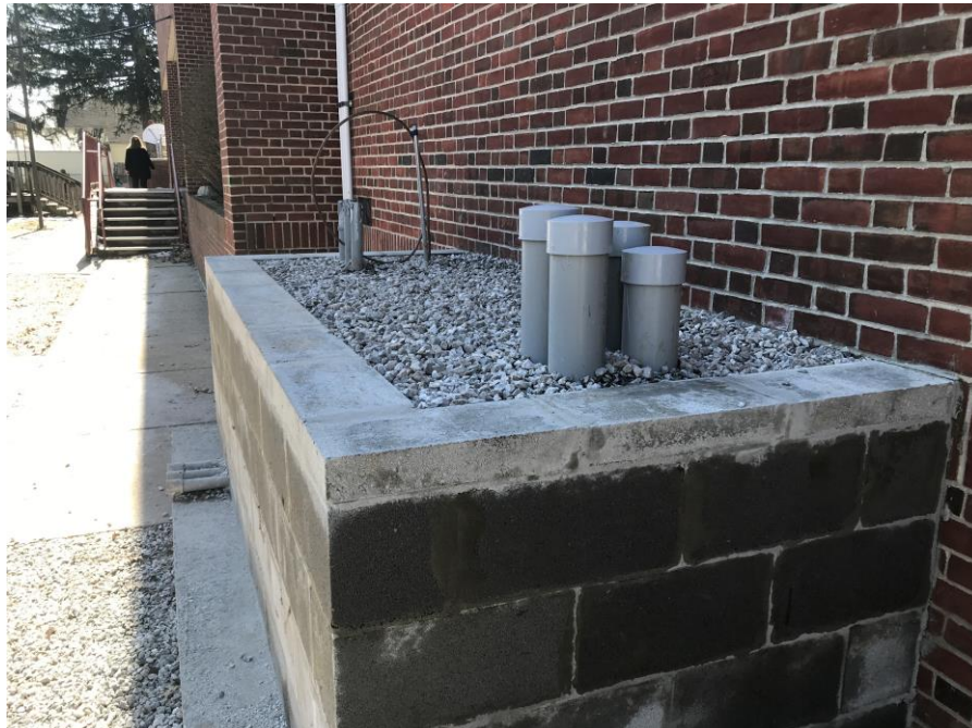
Preparation for slab for switchgear - Clinton Elementary School
