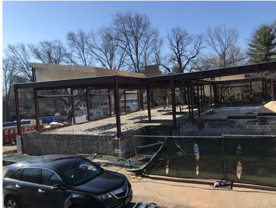
Closing metal framing and prep for SOG - Jefferson Elementary School
