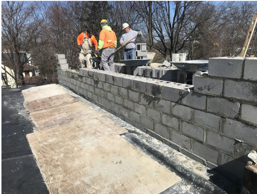
CMU Block parapet wall at area A - Clinton Elementary School
