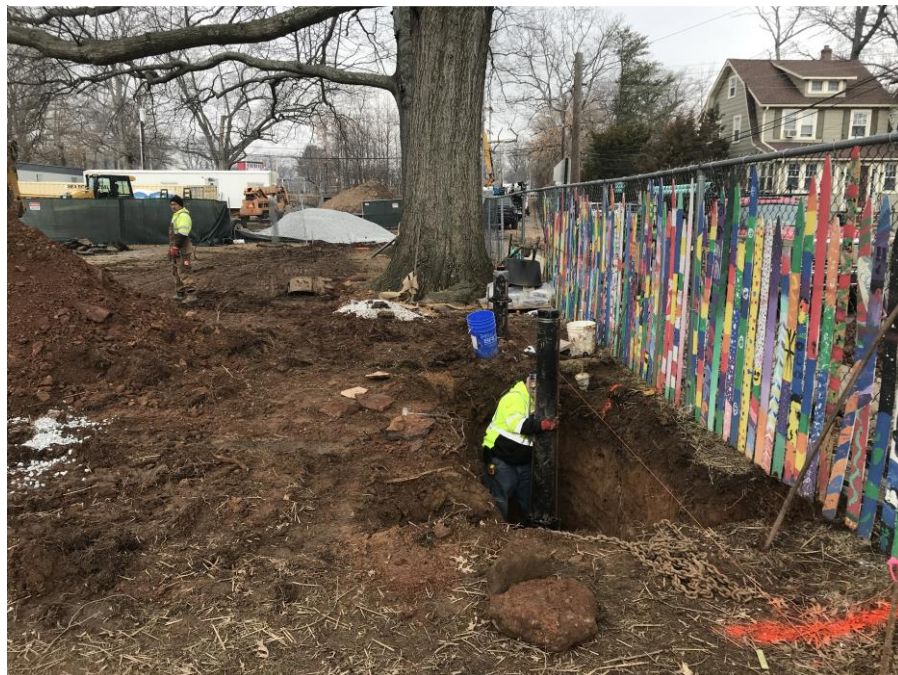
New Site Domestic and Fire lines underway - Clinton Elementary School
