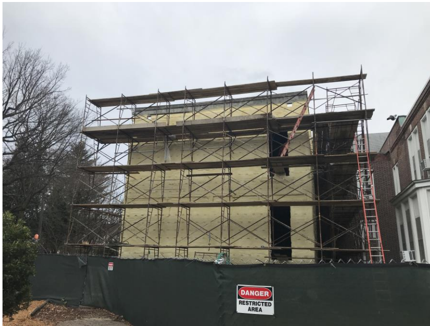
Spray on exterior insulation underway - Clinton Elementary School
