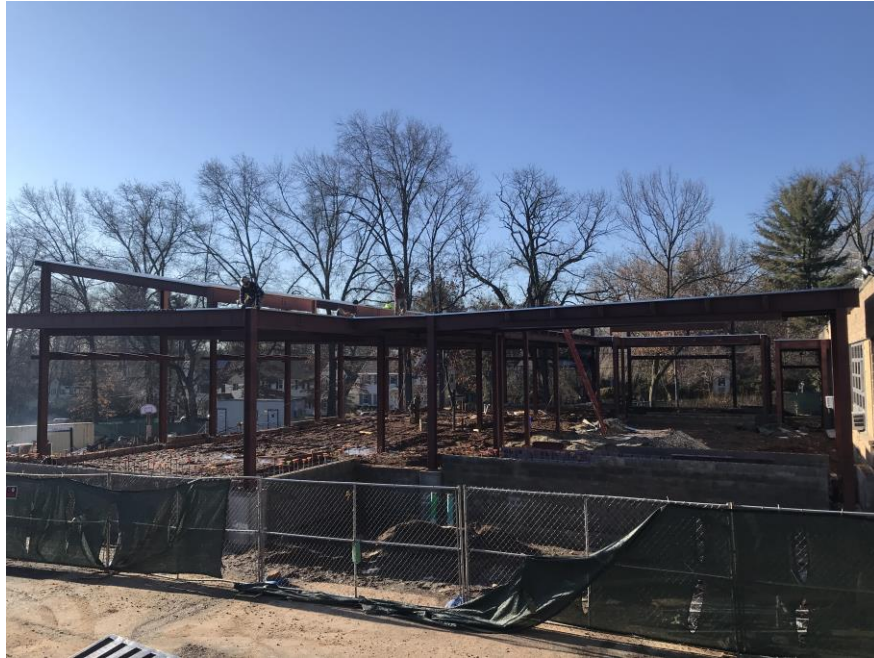
Roof metal welding underway - Jefferson Elementary School
