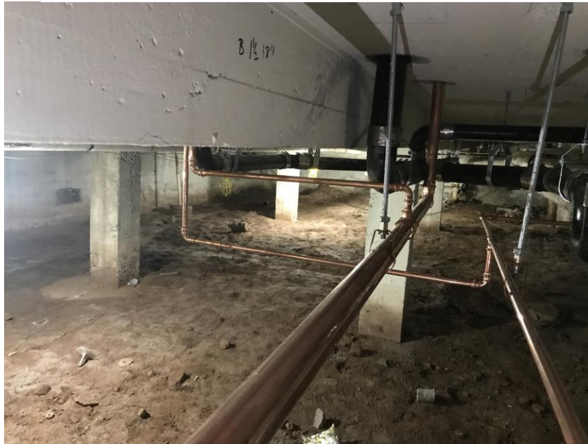
Water piping for new bathroom underway - Clinton Elementary School
