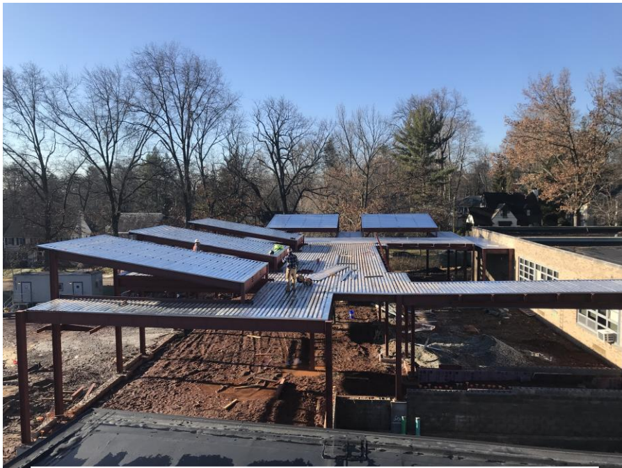
Steel metal deck underway - Jefferson Elementary School
