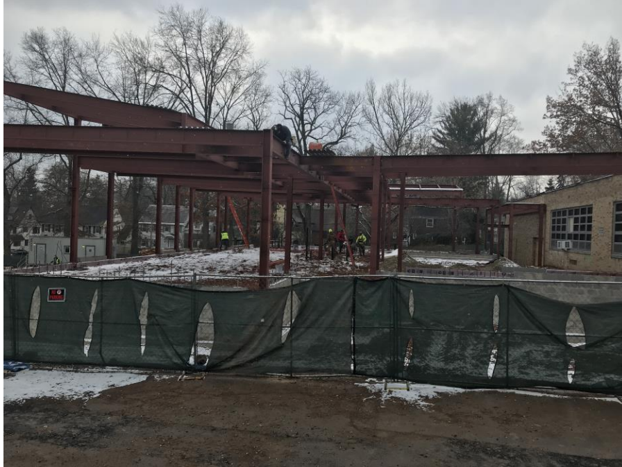
Steel erection underway - Jefferson Elementary School
