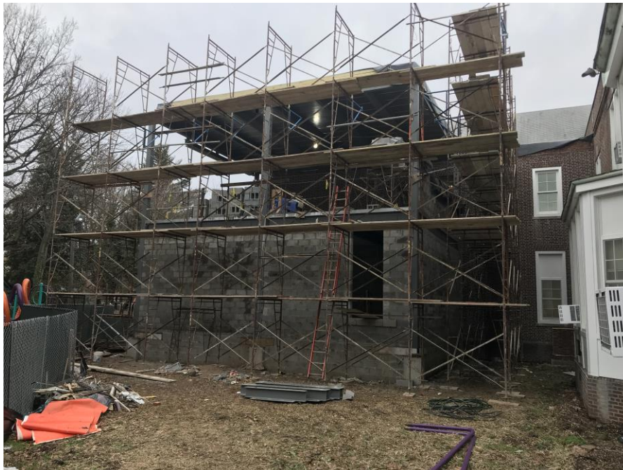
Set up scaffold at Area C - Clinton Elementary School
