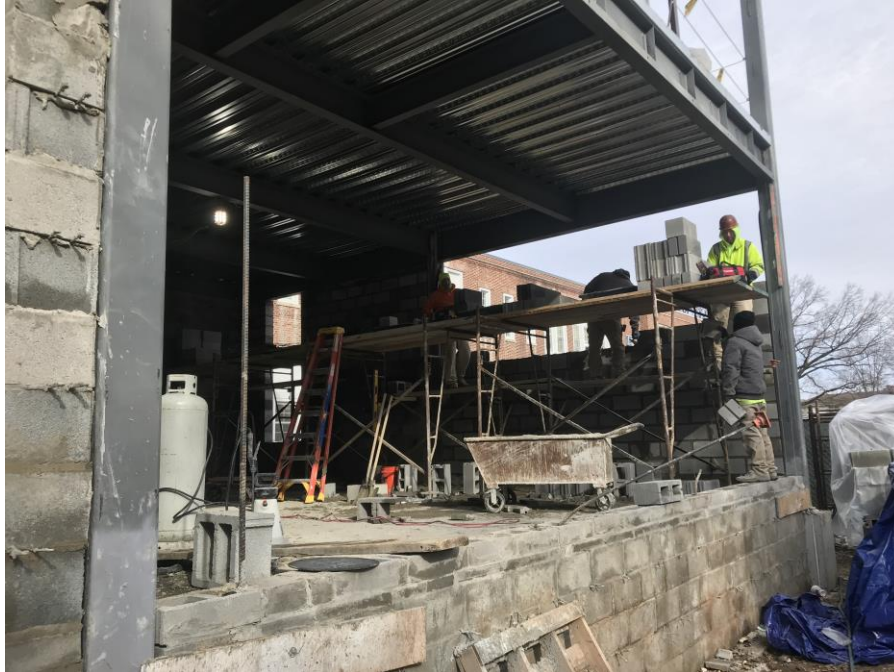
Masons working on Area C - Clinton Elementary School
