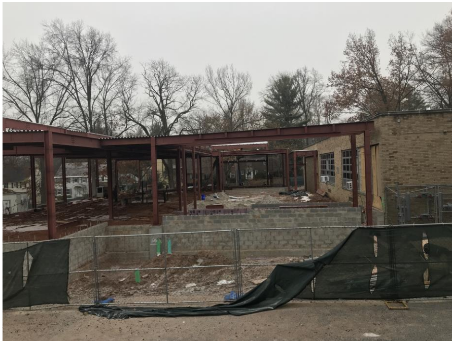
Roof metal deck underway - Jefferson Elementary School
