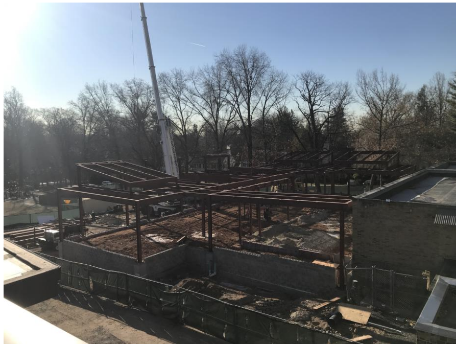
Steel erection underway - Jefferson Elementary School
