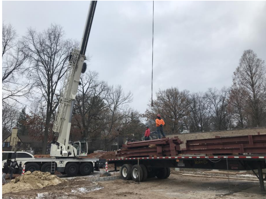
Steel Delivered to Jobsite - Jefferson Elementary School
