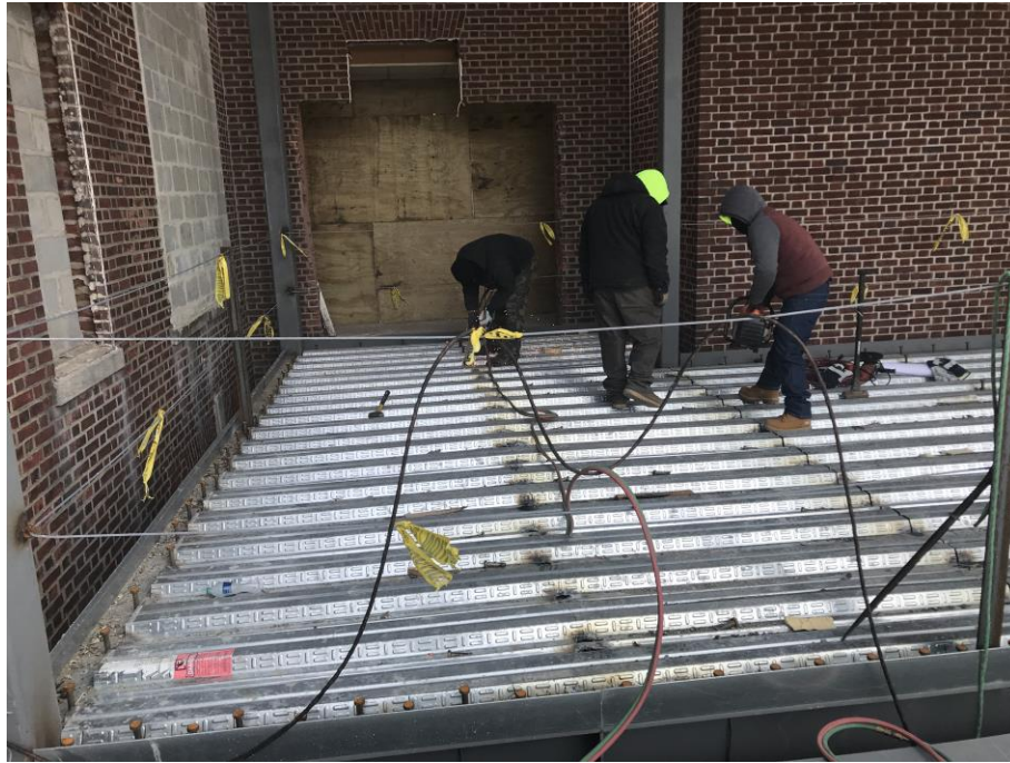
Ironworkers working at Area A metal Deck - Clinton Elementary School
