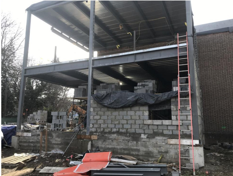
Area C CMU exterior wall underway - Clinton Elementary School
