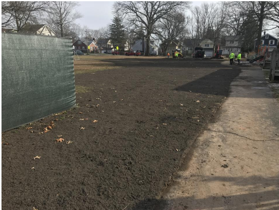
PSE&G site repairs - Clinton Elementary School
