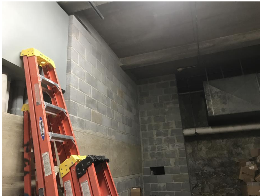
New CMU wall for Electrical Feeders - Jefferson Elementary School
