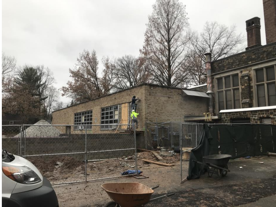
Existing exterior wall Demo - Jefferson Elementary School
