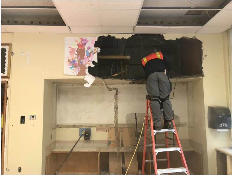
Demolition underway at Classroom A113 - Jefferson Elementary School
