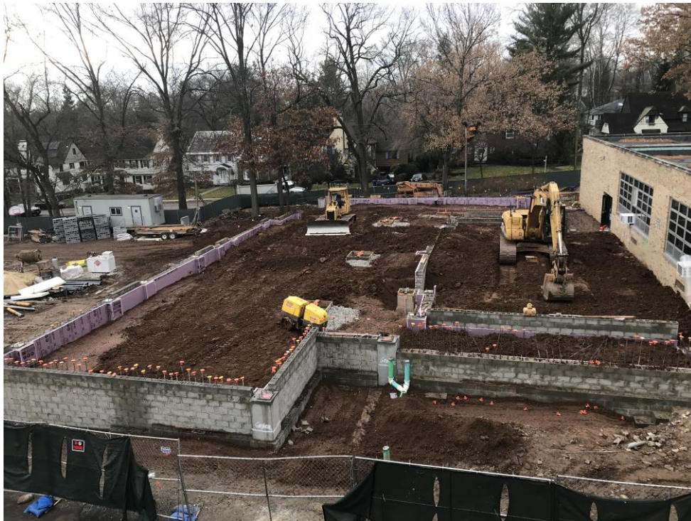
Backfill operations underway - Jefferson Elementary School
