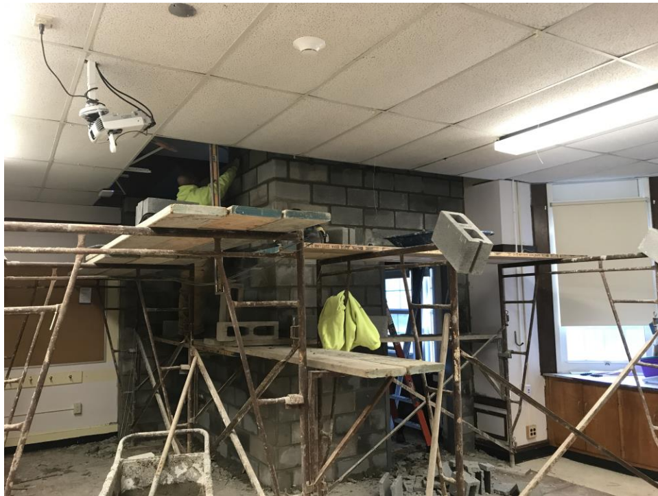
CMU Bathroom walls - Clinton Elementary School
