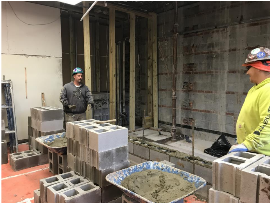
CMU Wall Partition at Classroom A113 - Jefferson Elementary School
