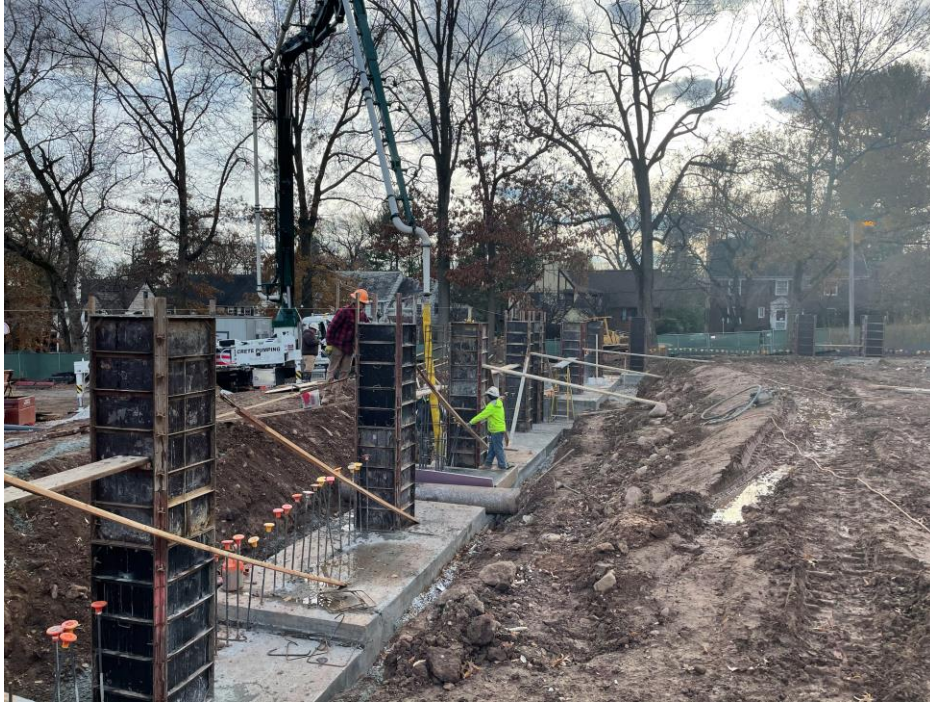
Pouring concrete Piers - Jefferson Elementary School
