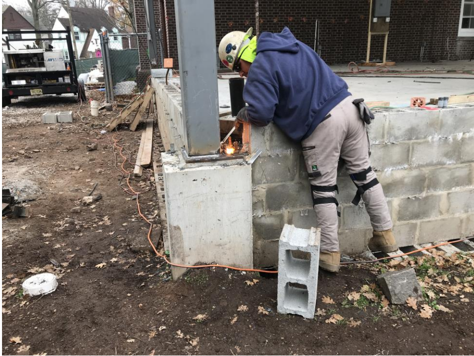
Steel Column Welding underway - Clinton Elementary
