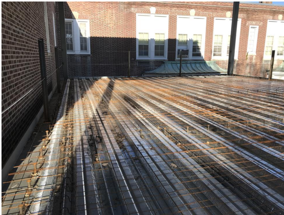
Slab on Deck Preparation at area C - Clinton Elementary School
