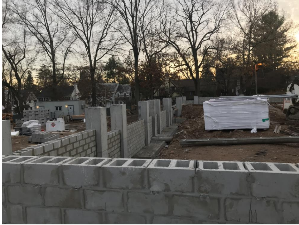
Foundations work underway - Jefferson Elementary School
