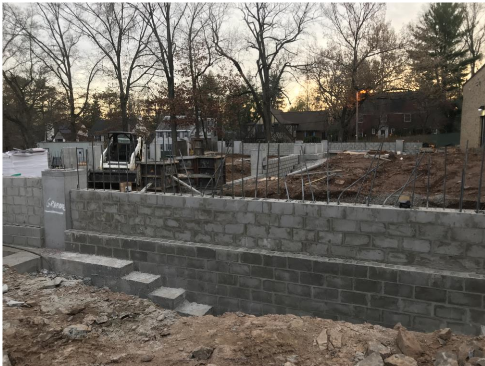
Backfilling underway - Jefferson Elementary School Epic Management, Inc.
