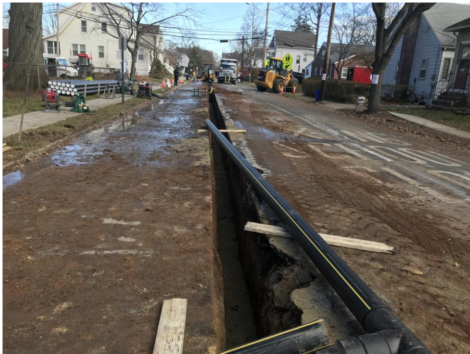
New Gas line - Clinton Elementary School
