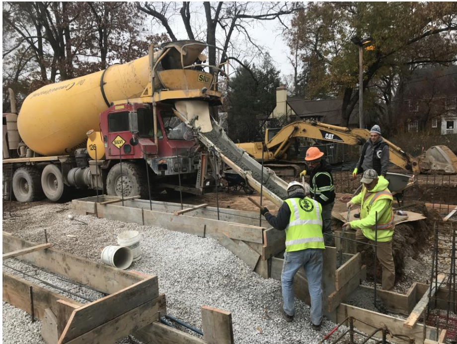
Poured footings - Jefferson Elementary School
