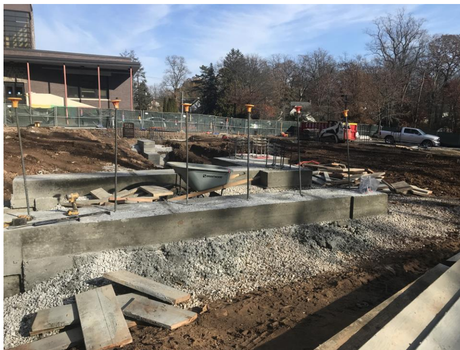
Concrete Footings Jefferson Elementary School
