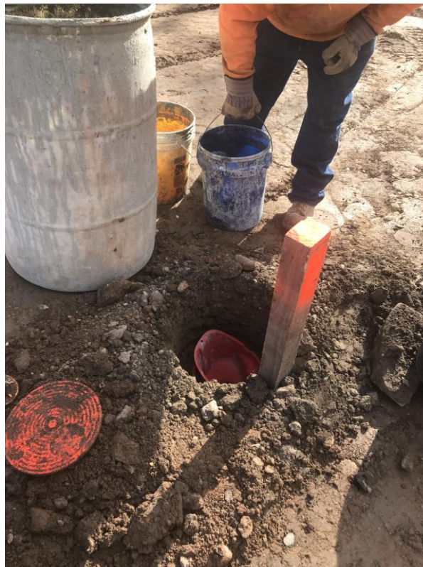
Closing and sealing existing Monitoring Well - Jefferson Elementary School
