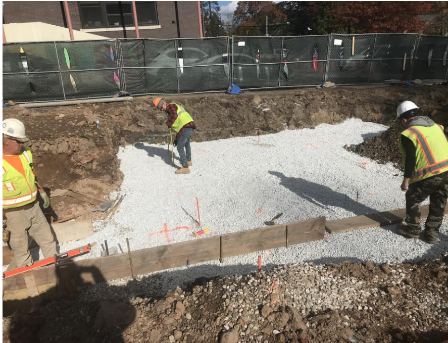
Setting forms for footing - Jefferson Elementary School
