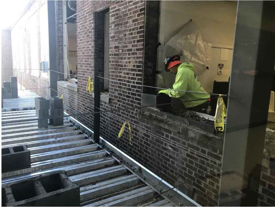
Masons infilling Window Opening – Clinton Elementary School
