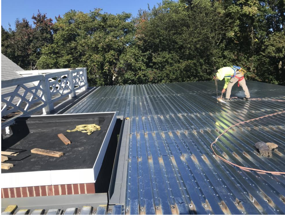
Installing Metal Deck at A – Clinton Elementary School
