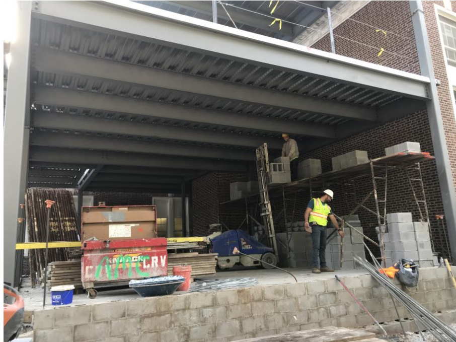
CMU block installation underway area A – Clinton Elementary School
