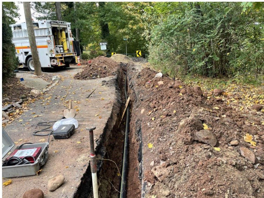
New Gas line underway - Jefferson Elementary School
