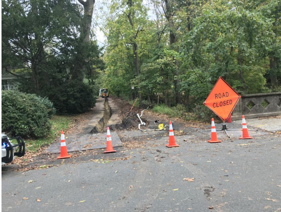
PSE&G new gas trench underway - Jefferson Elementary School
