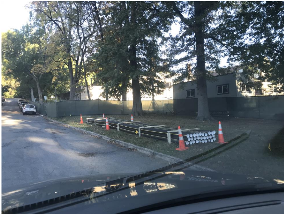
PSE&G gas piping delivered to site - Jefferson Elementary School
