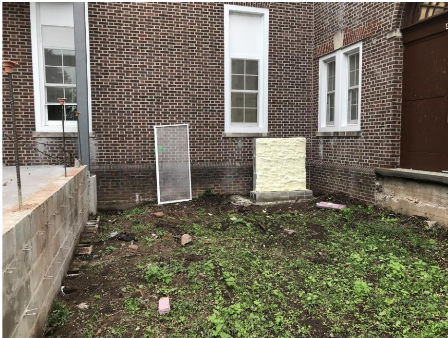
Masonry Mock up – Clinton Elementary School
