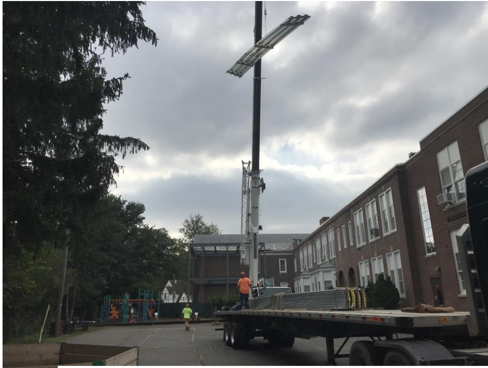
Crane erecting steel Metal Deck at C – Clinton Elementary School
