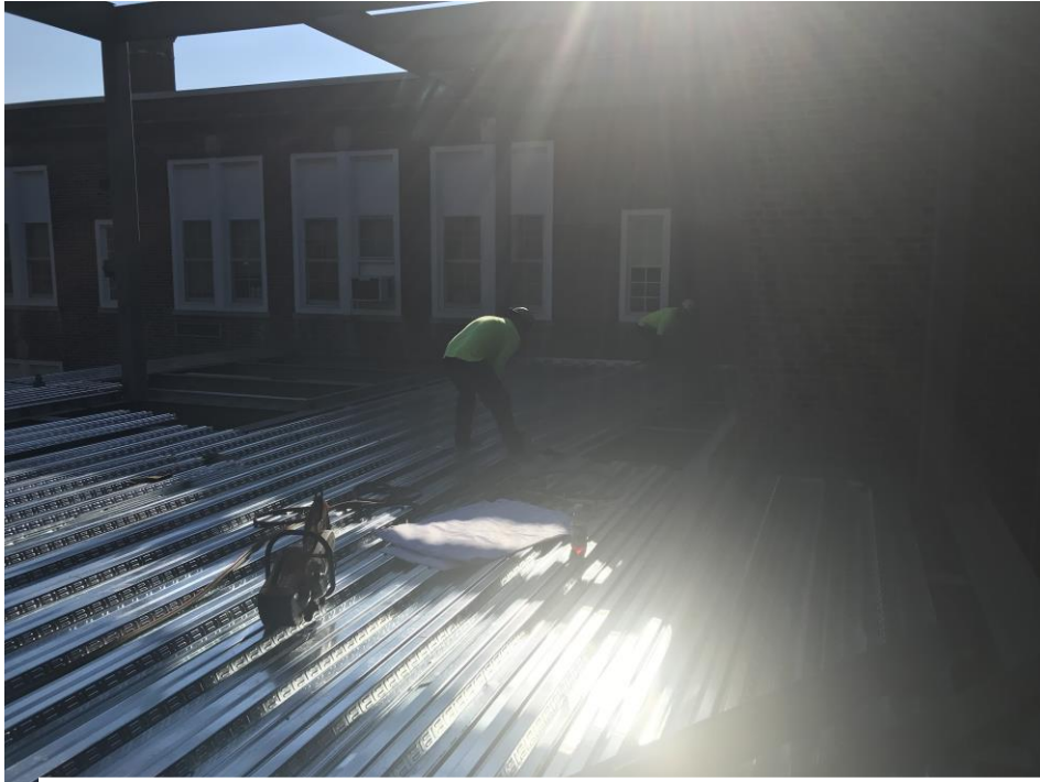
Metal Deck installation underway area A – Clinton Elementary School
