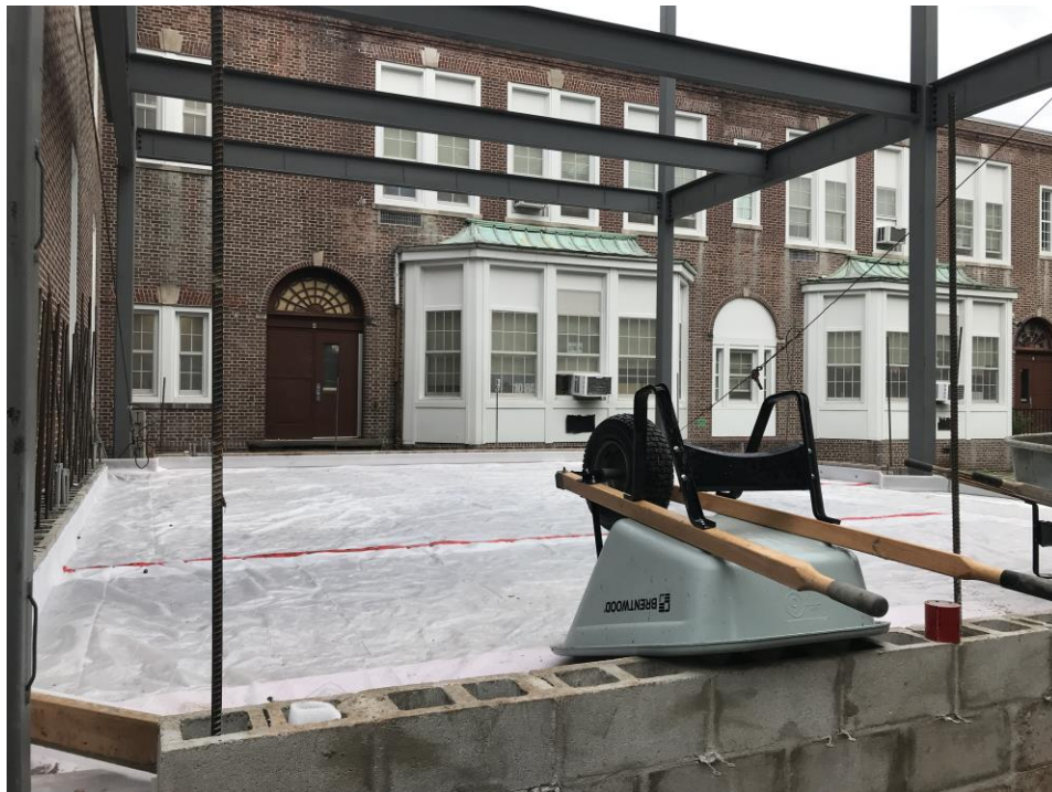
Slab on Grade Preparation at area C – Clinton Elementary School
