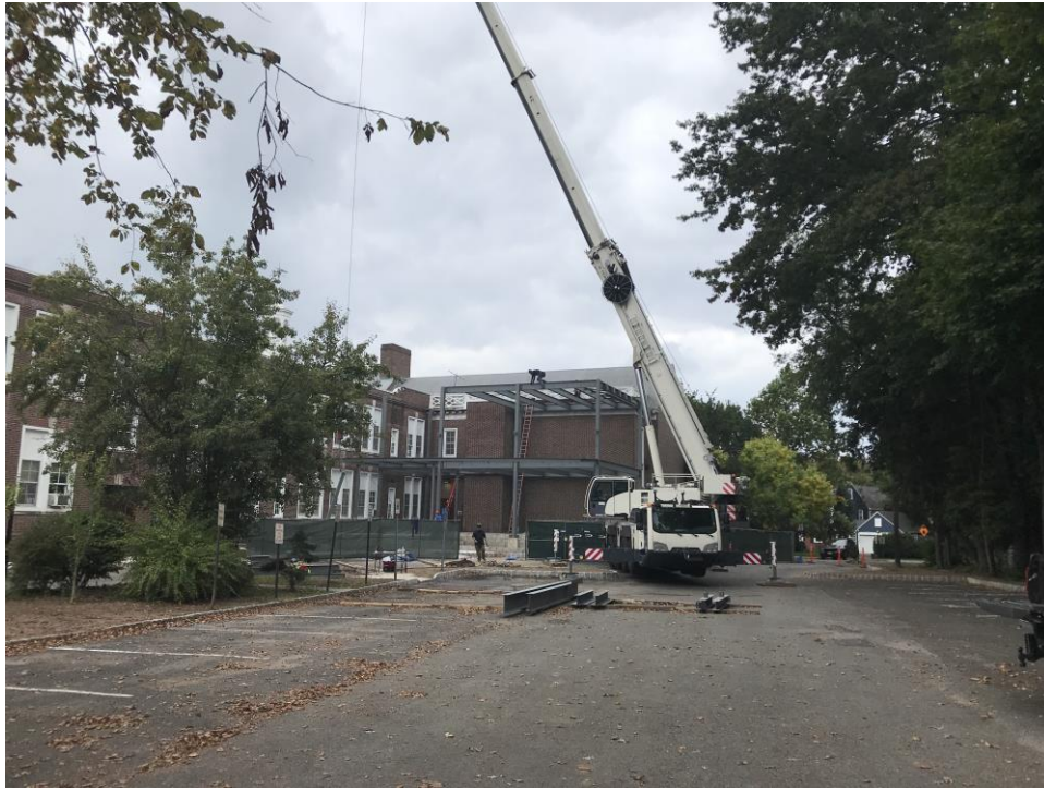
Steel erection at area A – Clinton Elementary School
