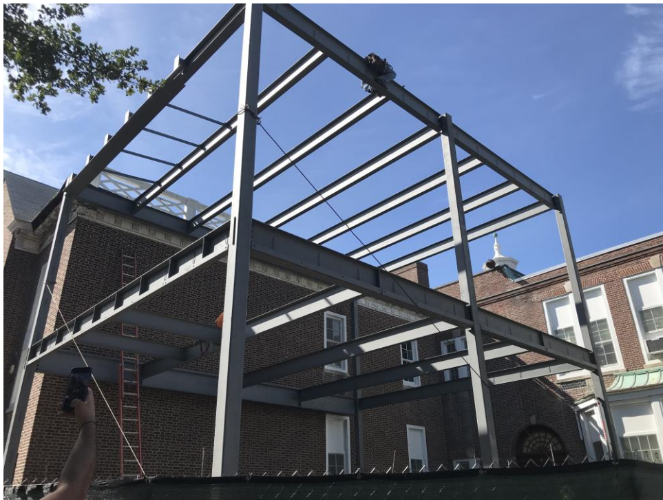
Steel erected at area C – Clinton Elementary School
