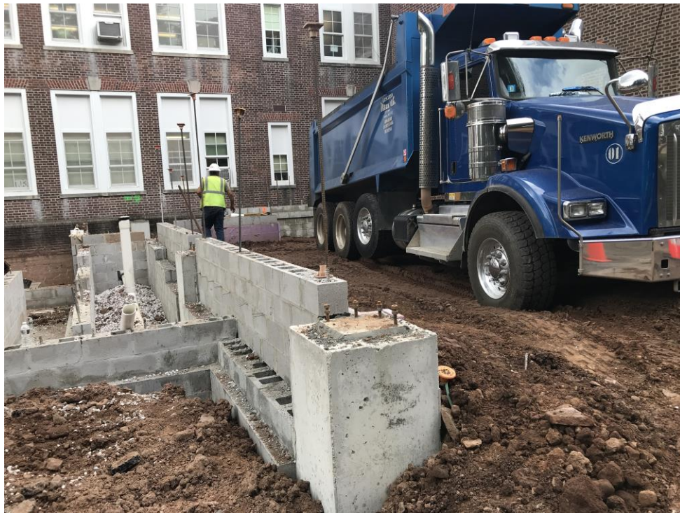
Backfill area at new Addition A – Clinton Elementary School
