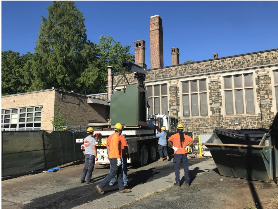
New Transformer and Pad Delivery – Jefferson Elementary School
