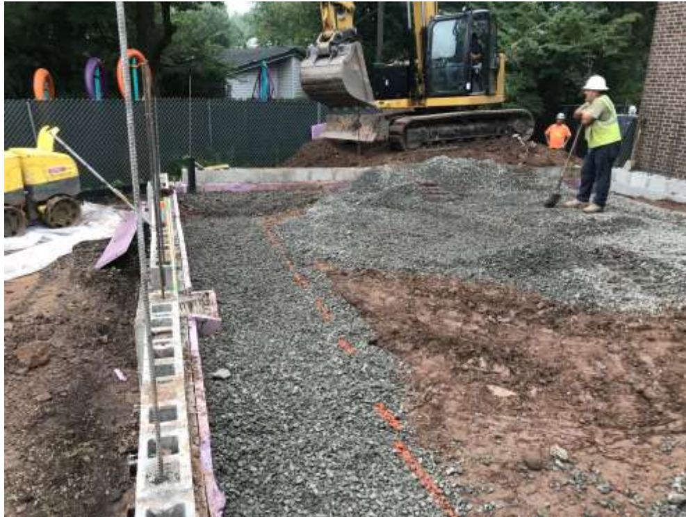
Area C back filled : Clinton Elementary School
