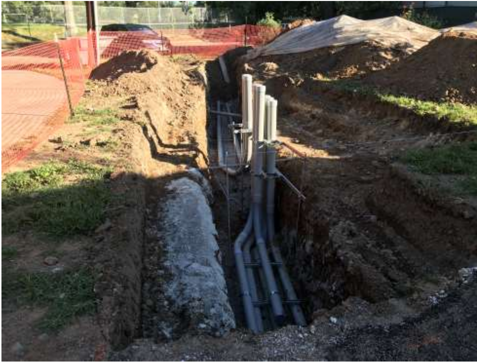
Excavated for New transformer / pole – Clinton Elementary School
