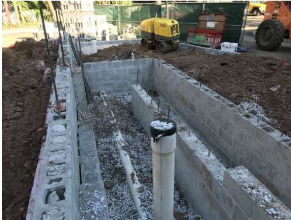
Front Entrance Ramp Area foundation: Clinton Elementary School
