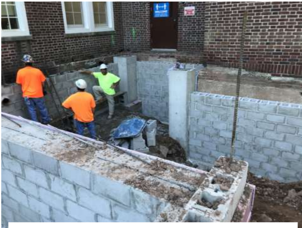
Foundation work –Clinton Elementary School
