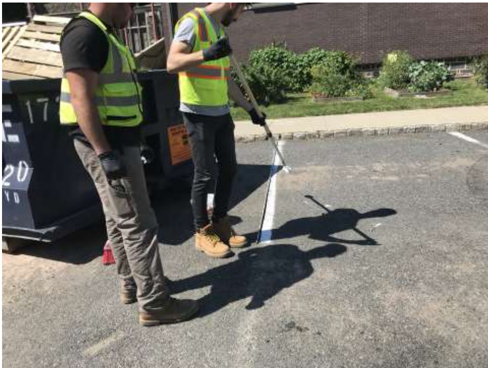
Temporary parking lot line striping -Jefferson Elementary School
