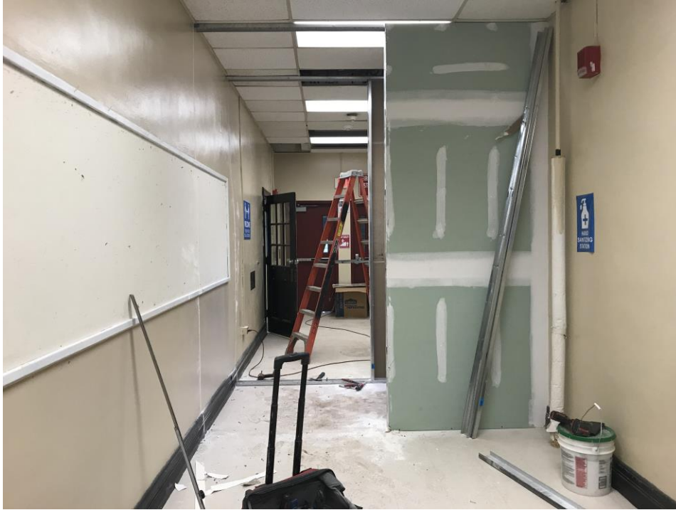
Modifying temporary partition – Clinton Elementary School
