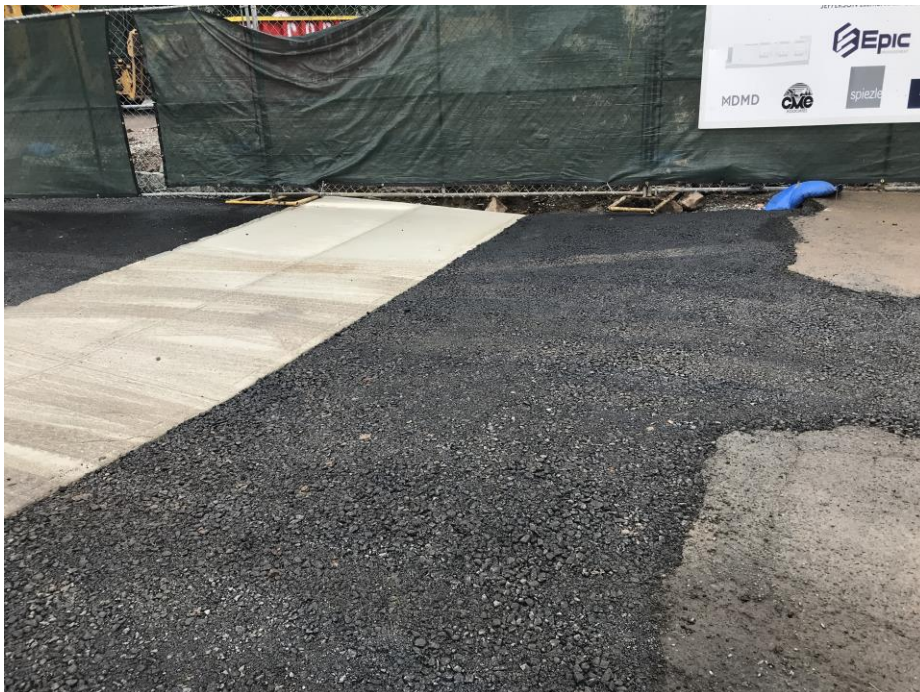
Paved access entrance to dumpster location -Jefferson Elementary School
