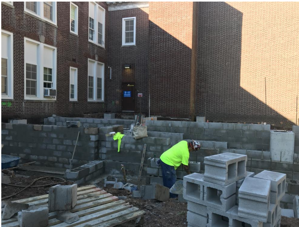
Foundation work at New Main Office – Clinton Elementary School
