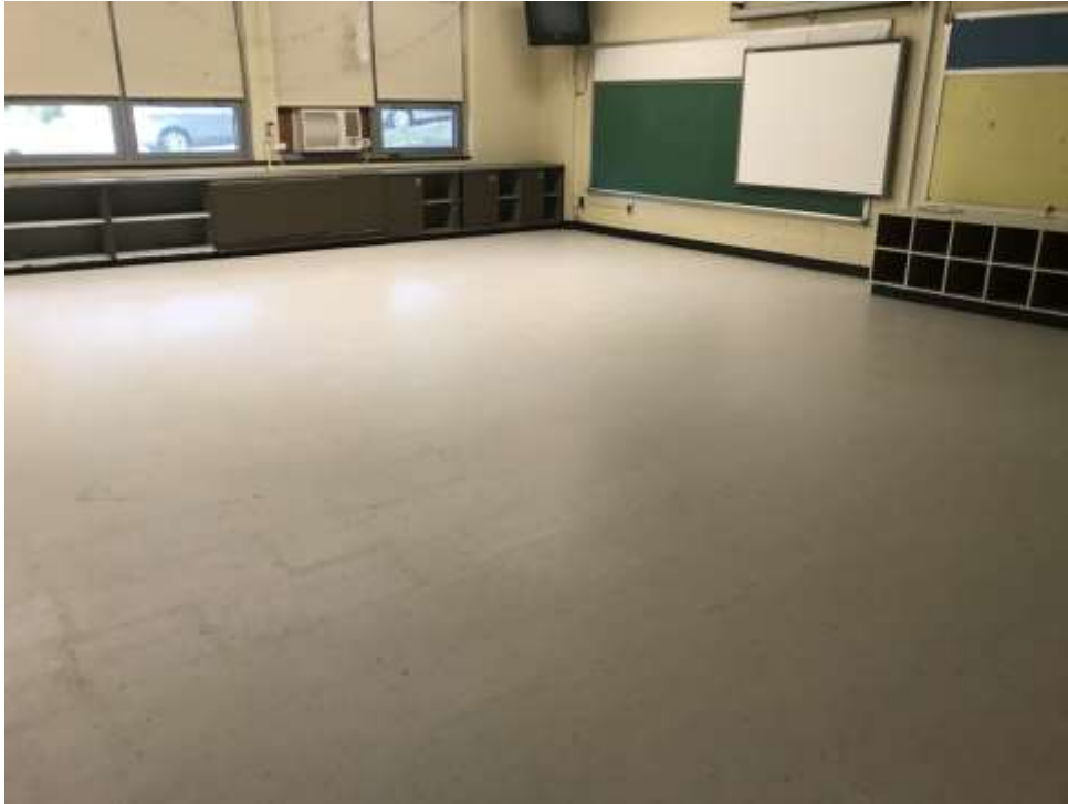
New VCT floors – Jefferson Elementary School
