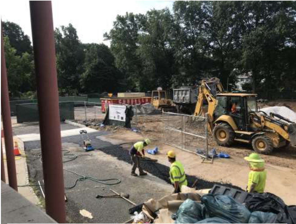
Paving Primary Feeders to Transformer – Jefferson Elementary School
