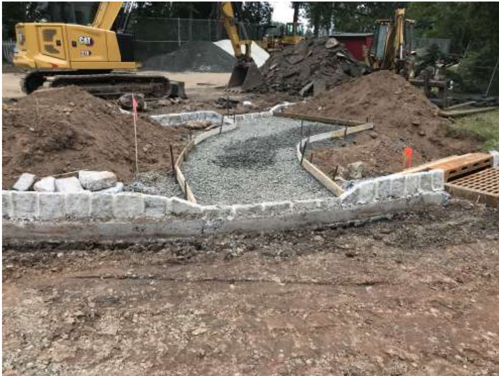
Site Work preparation – Clinton Elementary School
