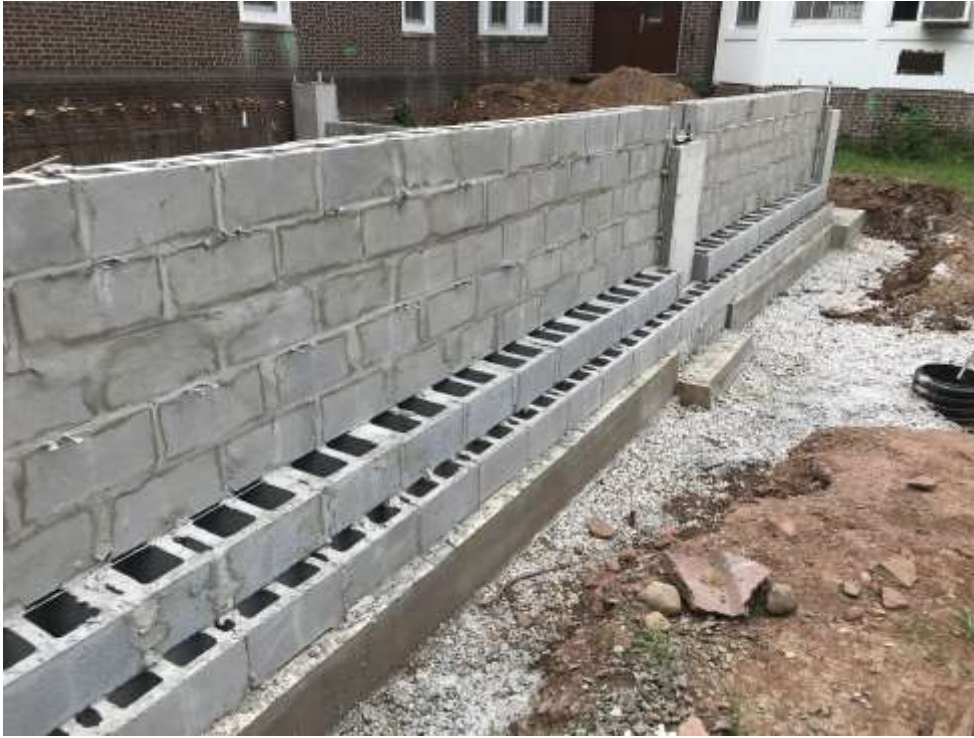
Foundation C– Clinton Elementary School
